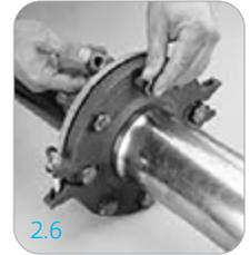
**Note:** Take care to assure that the gasket lip is not bent backwards or pinched between the two flanges.
