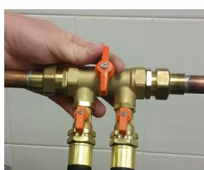
7) Set system fill and purge valve to allow flow in and out of pump cart.
