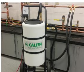
10) Let fluid circulate to fill system and purge air, check for air entering tank at bottom of return dip tube, maintain fluid levels.
