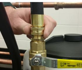
2) Connect opposite end of hose to pump cart supply at ball valve.
