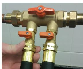
3) Connect second hose to fill and purge valve outlet.
