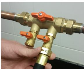
1) Connect hose to fill and purge valve inlet.
