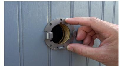
Step 4: Tab with hole positioned at 6 o'clock
