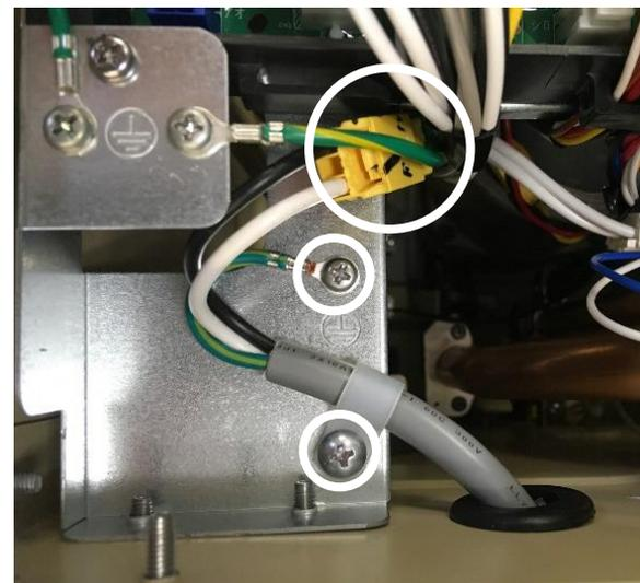
3. Pull grommet and cord through bottom of water heater cabinet.
