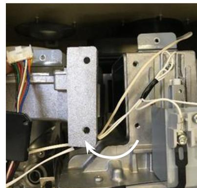
**NOTE:** Be careful not to damage the plastic Heat exchanger elbow in front of the orifice block when removing the blower assembly.
