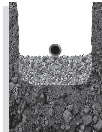
Trench in poor soil
