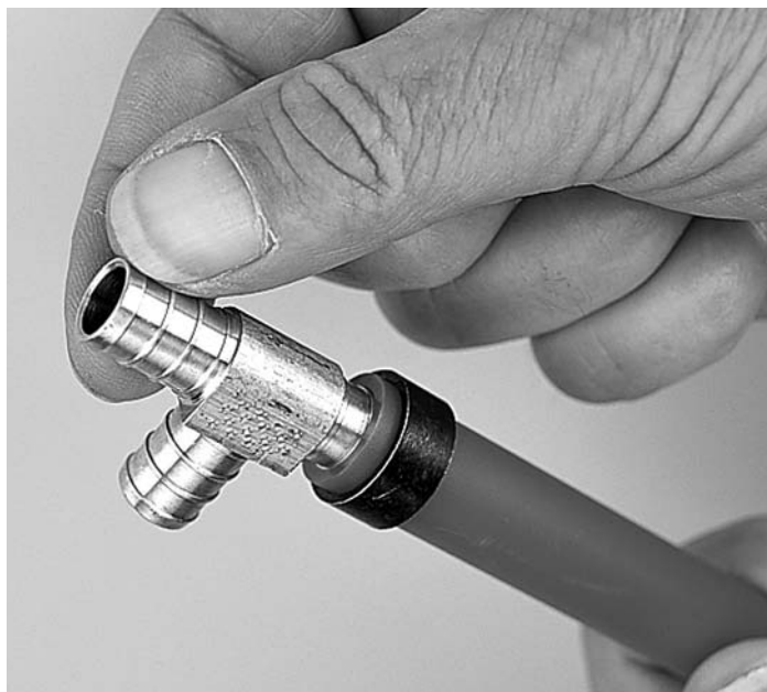
1. Position the crimp ring and insert the fitting into the tubing.
