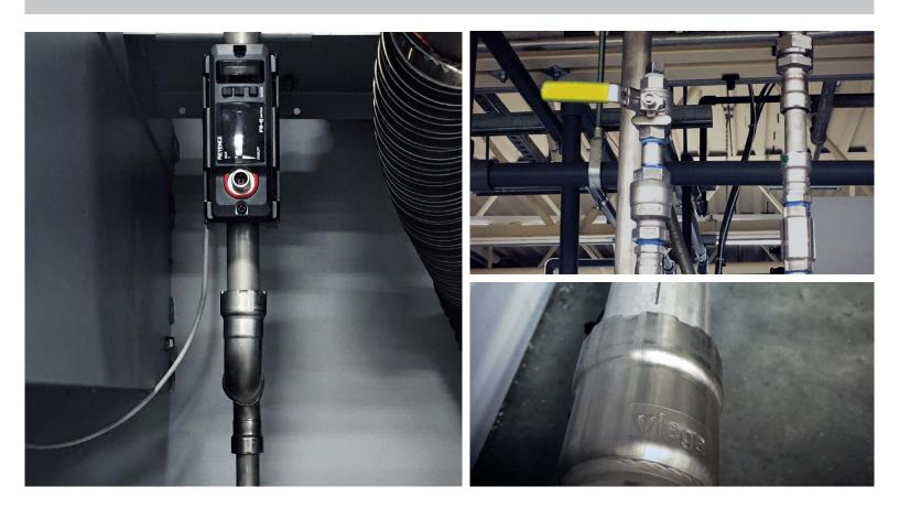
In Lewiston, Idaho, Mike's Mechanical installed MegaPress Stainless fittings in a high-tech facility manufacturing circuit boards for a broad range of products. During production, the boards are cleaned using high heat and corrosive chemicals, so the use of stainless steel pipe and fittings was essential.
