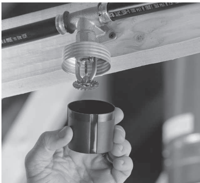
Keep heads within protective shell during installation
