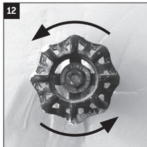
13. Once the water has stopped sputtering as the air has been bled from the line, shut off the previously opened faucet from step 2.
