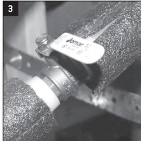
4. Install the FloodStop Valve between the rigid water line coming from the manual cold-water valve and the water heater, positioned so that the arrow on the side of the valve is pointing toward the water heater (in the direction of the flow of water.) **NOTE:** The FloodStop Valve should be installed within 2 feet of the water heater so that the Leak Sensor can lay flat on the floor.
