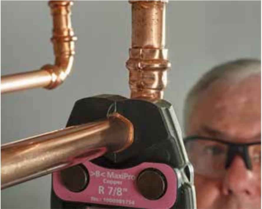
**Note:** When using a press tool, wear ear and eye protection.
