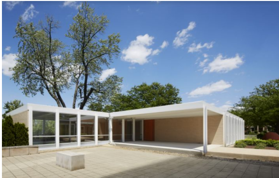
Exterior of McCormick House (2018). Kendall McCaugherty © Hall+Merrick Photographers
