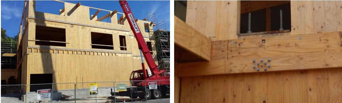
Figure 2.11 Kaikoura District Council Building under construction; wall-to-beam connection with a ring of bolts
