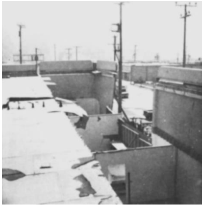
a) Vector Electronics Building, Sylmar, CA Collapsed roof due to failure of support
