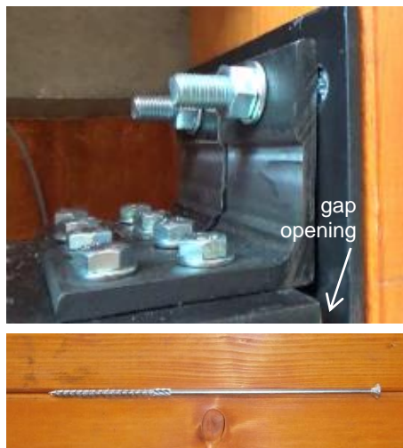
Figure 8.22 Beam-column-joint gap opening (top) and undamaged fastener of the diaphragm connection to the secondary beam (bottom)
