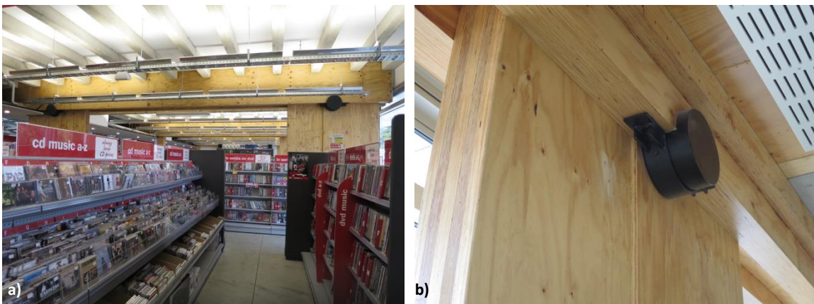
Figure 2.12 The Warehouse building in Richmond with wall-to-beam connection via a large diameter pin
