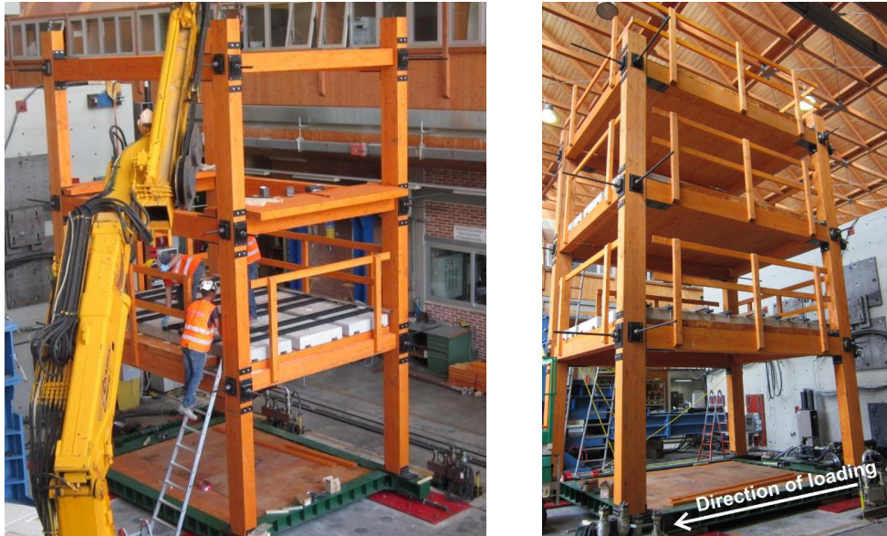
Figure 8.18 Experimental setup of the 3 storey post-tensioned glulam frame building
