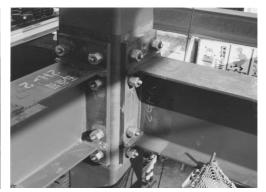
(a) A splice joint in a double chord truss where the bolts (loaded in shear) have been tightened with the aid of access holes
