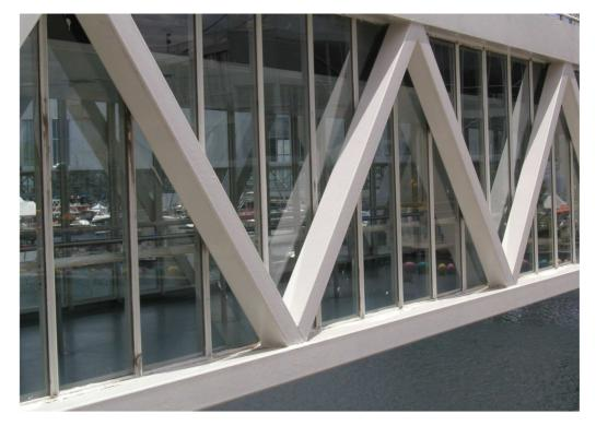
Truss with 100% overlapped joint
