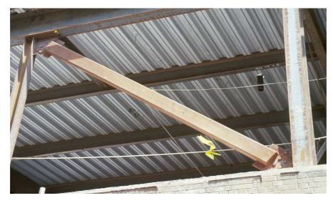
Figure 7.4 - Gusset plates slotted into a diagonal RHS bracing member, in a braced steel frame
