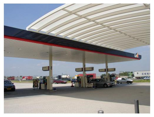
Figure 2.2 - Rectangular hollow sections used in the roof and for the columns of a petrol station
