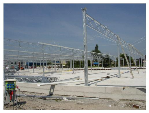
Figure 2.6 – Rectangular hollow section columns and trusses used in a glass house
