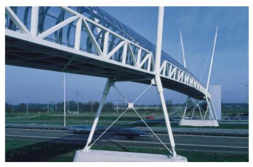
Figure 2.3 – Rectangular hollow sections used in a truss of a footbridge
