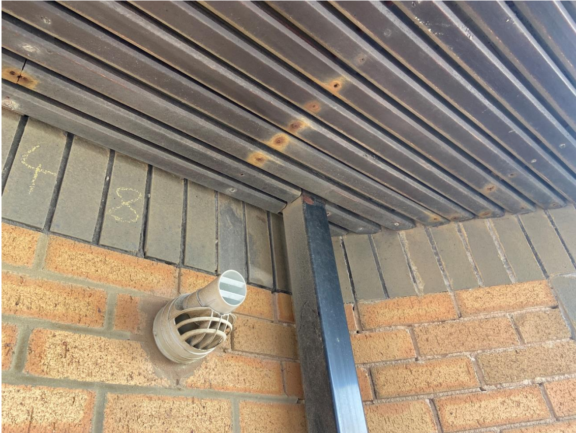
3. Corroding fixings to existing timber slats
