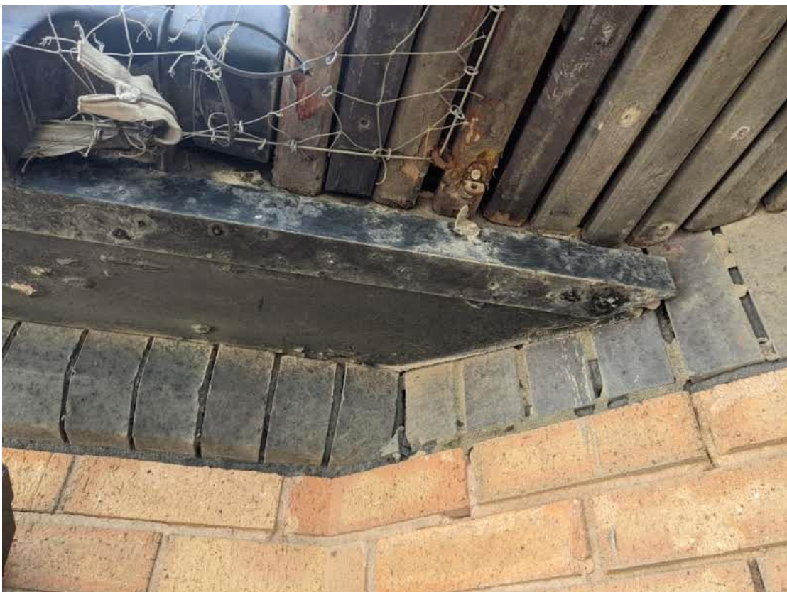
4. Timber slats generally in poor condition
