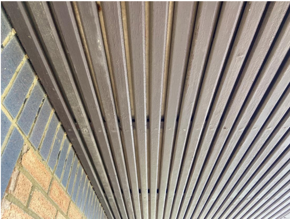
1. Typical timber slats to underside of balcony
