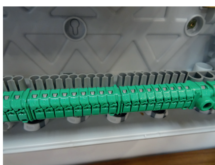
Earth terminal block: automatic connection
