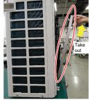
5) Disassemble the front cabinet ass'y.(5 screws in front side, 4 screws in right side.)
