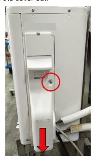
2) Remove the screw fixing Terminal Cover and Cord Clamp, then take them out.
