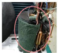
(Method of remove compressor cover)
