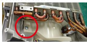
25) Remove 2 screws fixing Side Cover L.
