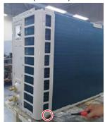
7) Disassemble side cover L.(6 screws)
