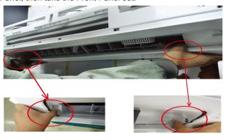
8) Cut the Wire Fixing Band and remove the Thermistor. (CLC6001i-W 25/35 E, CLC6101i-W 50 HE)
