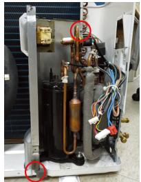
12) Remove the screw fixing Motor Angle, then take it out.
