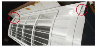
Lift the Open Panel up, then Slide the Open Panel' Hook along the Guide to remove it (right and left side).
