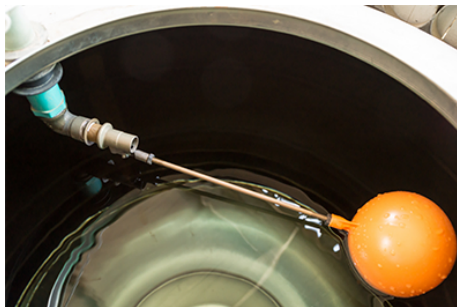
Level control float switch
