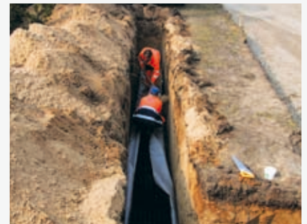
Faskine under etablering
