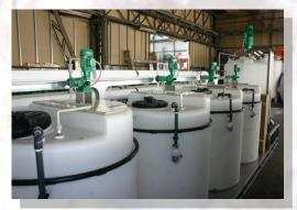
Acids dosing units, eventually managed by proper on line instruments, relevant management software dgestione.
