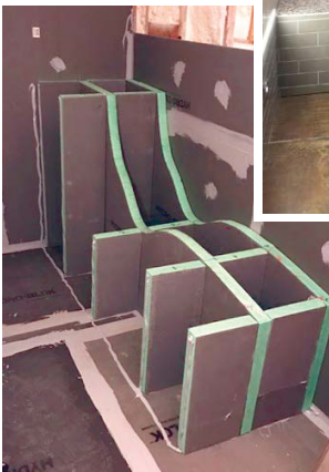
Custom shower benches created with HYDRO-BLOK 2" Building Board with dual Linear Drains and floor insulation for a Commercial Steam room project.
