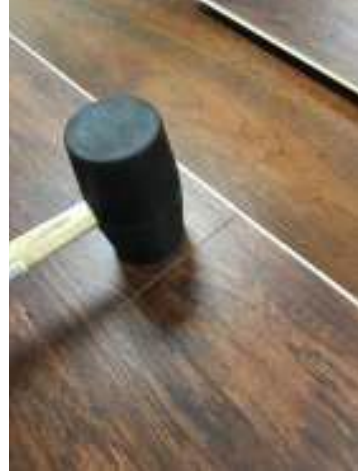
Correct (1/2" to 1" away from seam)
