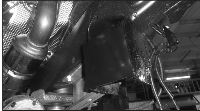
FIGURE 23 - SHOWN ALREADY PAINTED
