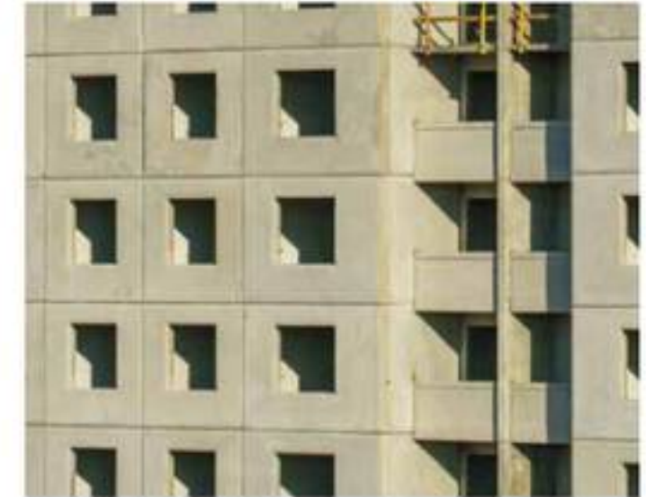
In an industry-first practice, damp proofing done to ensure no seepage or dampness.
