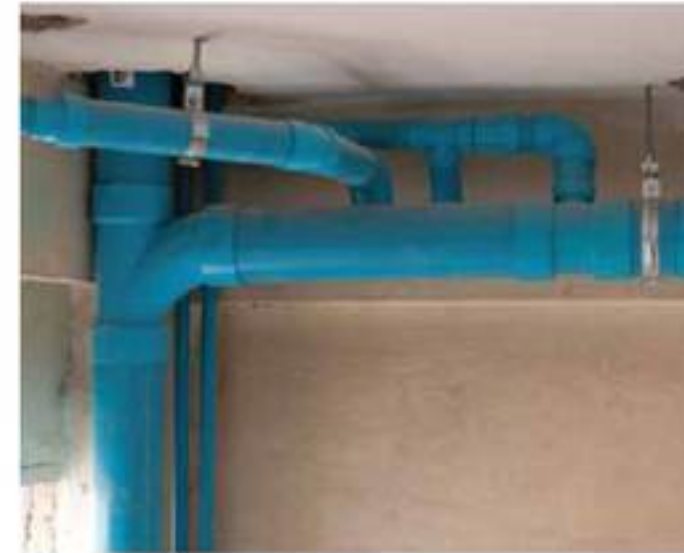
Provision of concealed secondary drain spout to drain accidentally seeped water.
