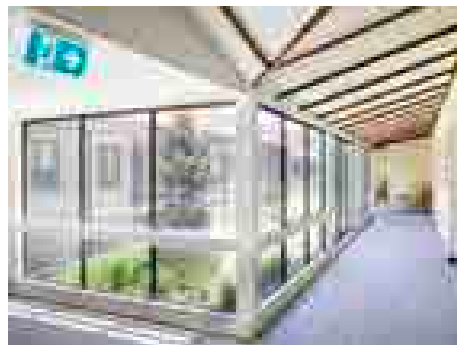
KOOROOTANG COURT RETIREMENT VILLAGE – COMMUNITY CENTRE AND LODGE BUILDING CORRIDOR REFURBISHMENT LENLEASE RETIREMENT LIVING IN COLLABORATION WITH ARKEE CREATIVE
