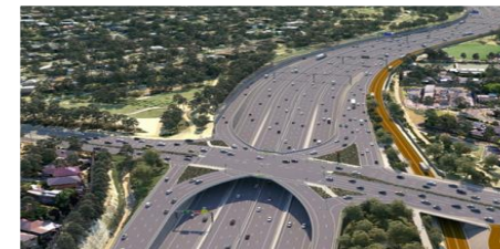
North-East Link Total Investment $20.6bn Completion target: 2028 Allowing Melbourne’s most populous suburbs in the south-east to be services from Melbourne’s North
