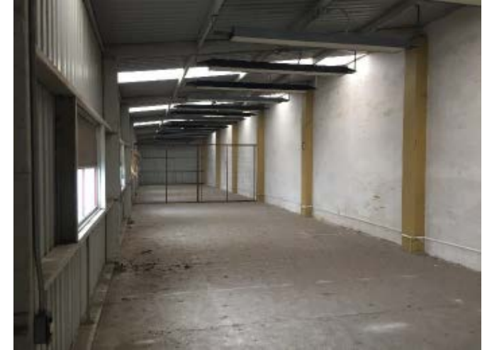
Nave industrial (interior)
