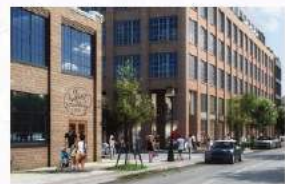
SHIRT FACTORY LOFTS Year Built: 2021 Type: Multifamily Units / Keys: 122
