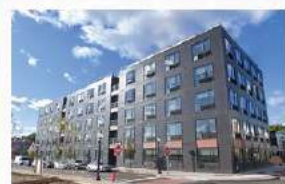
SONO 19 DAY Year Built: 2017 Type: Multifamily Units / Keys: 58
