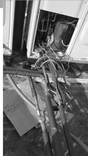
In modular systems all piping must be parallel with the units, these images are improper installation
