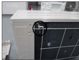
Outdoor Ambient Temp Sensor
