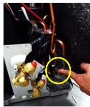
Condenser Temperature Sensor
