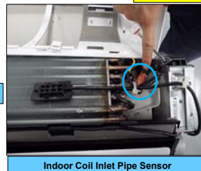
Indoor Coil Inlet Pipe Sensor
