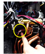
Compressor Discharge Temperature Sensor
