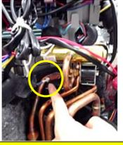
**Compressor Discharge Temperature Sensor**
