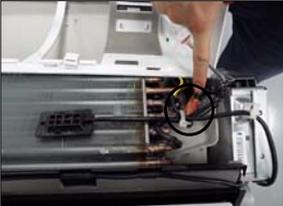
**Indoor Coil Inlet Pipe Sensor**
