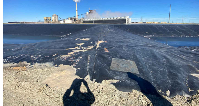
2709 - Facing North. Ash Pond B and South Equalization Basin Splitter Dike.
