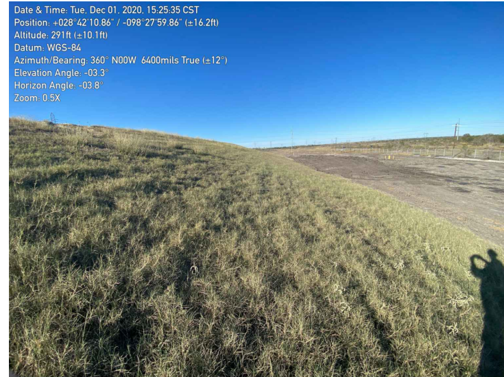
2908 - Facing North. East Exterior Slope, Interceptor Trench Construction in Background - Right Side.
