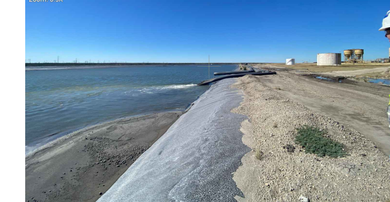
2775 - Facing West. Ash Pond A Dike Crest and Interior Slope.
