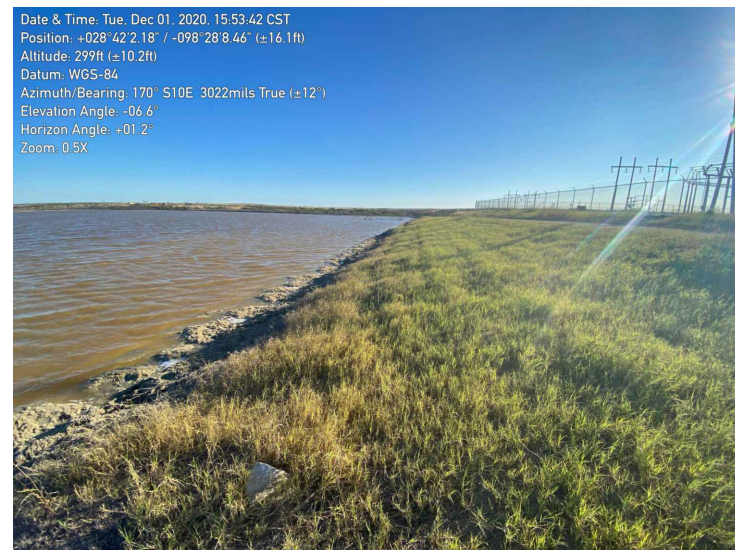
2981 - Facing South. Southwest Interior Slope.
