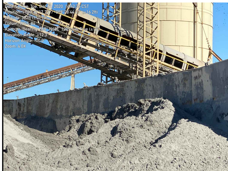
2889 - Facing Northeast. Ash Pile and Wall.
