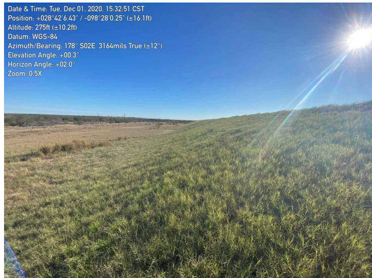
2916 - Facing South. Southeast Exterior Slope.
