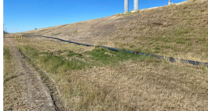
2699 - Facing Northwest. Ash Pond B, Exterior Slope.
