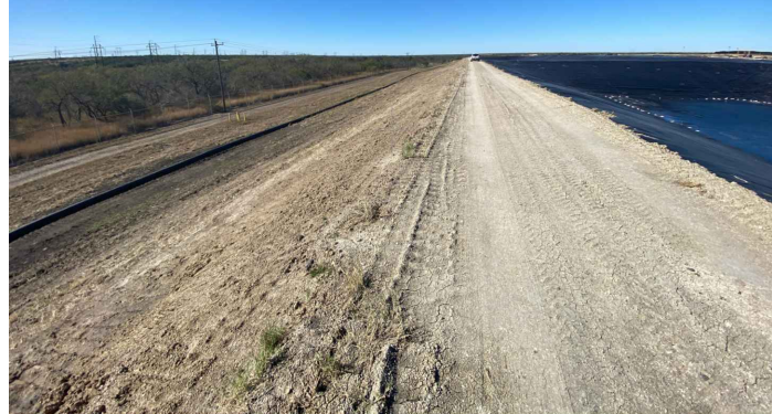
2706 - Facing West. Ash Pond B Exterior Slope and Dike Crest.
