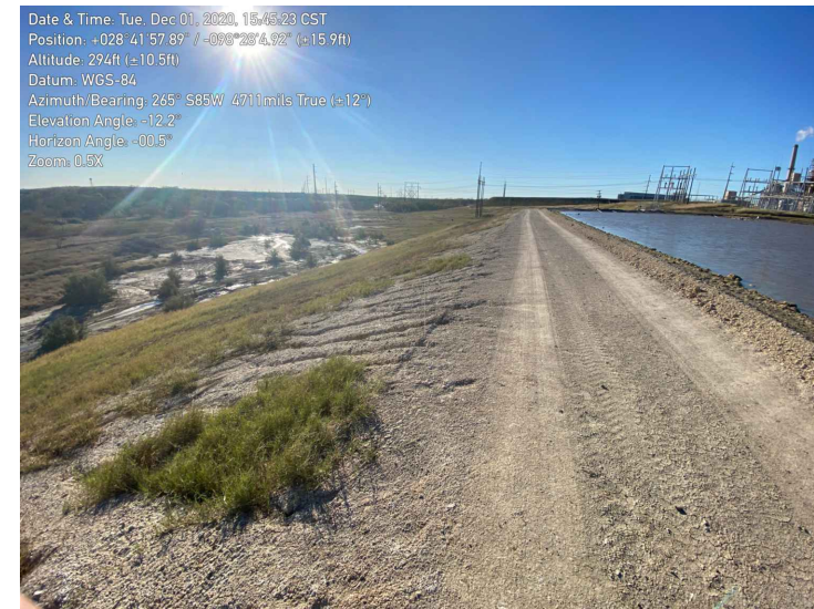
2953 - Facing West. South Dike Crest and Exterior Slope.
