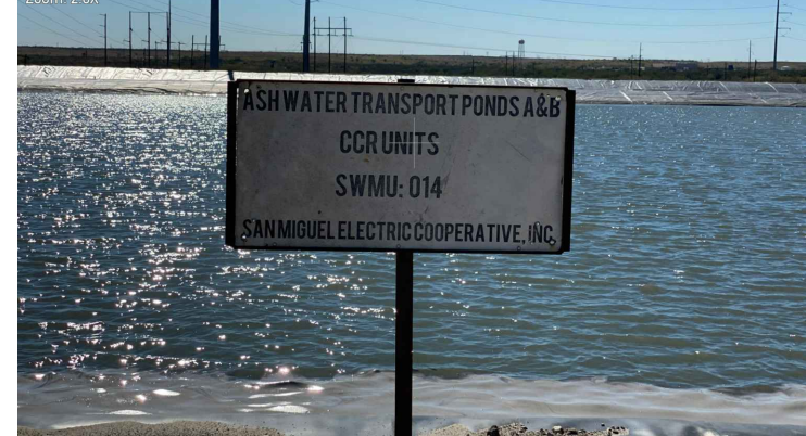
2778 - Facing South. Ash Pond A and Signage.
