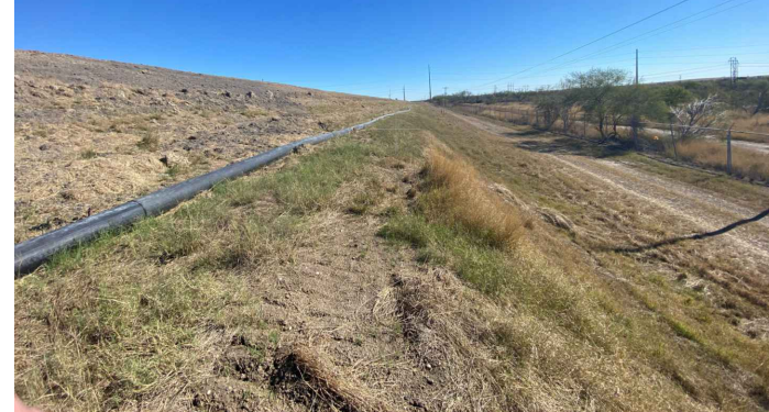
2717 - Facing East. South Equalization Basin Exterior Slope.
