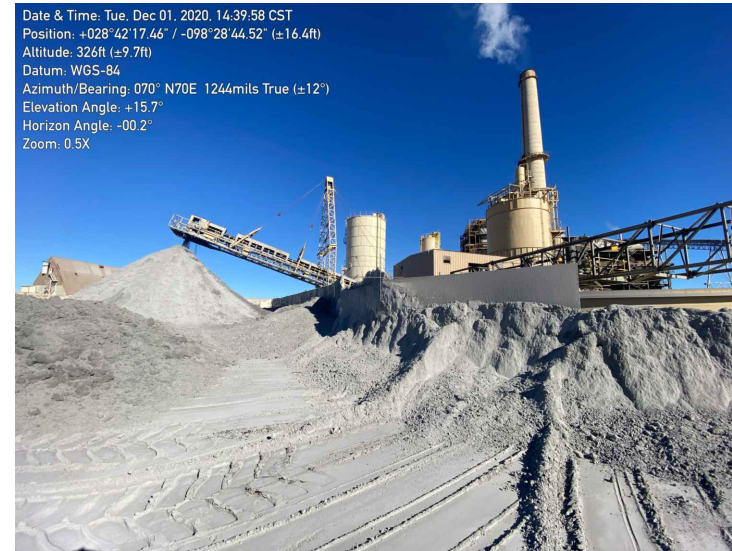
2883 - Facing Northeast. Ash Pile and Wall.
