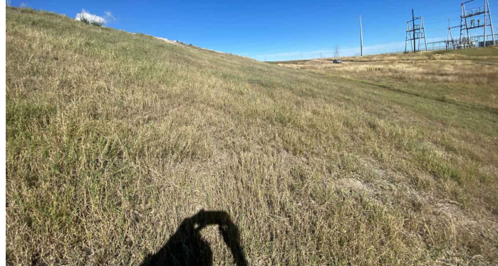
2677 - Facing North. A/B Ponds Exterior Slope.
