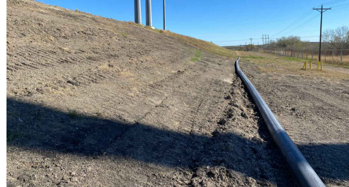
2702 - Facing East. Ash Pond B, Exterior Slope.
