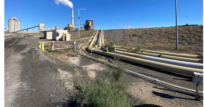
2730 - Facing Northeast. Ash Pond A, West Exterior Slope
