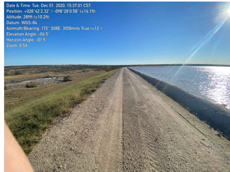
2935 - Facing South. Southeast Dike Crest.
