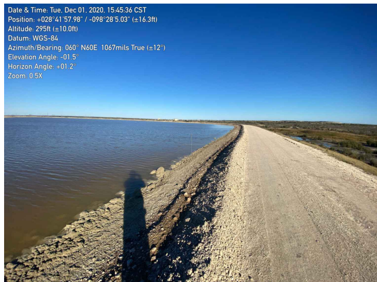
2955 - Facing East. South Dike Crest and Interior.
