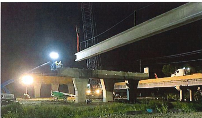
Placing beams at Parvin Branch Creek
