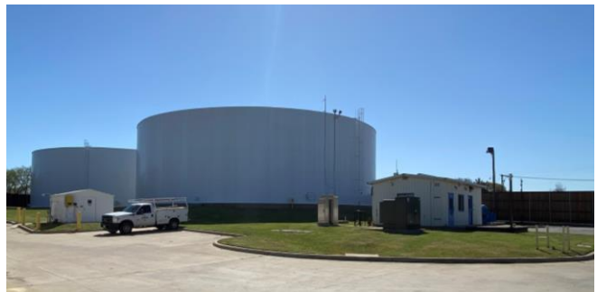
Figure 2.5. District Pump Station
