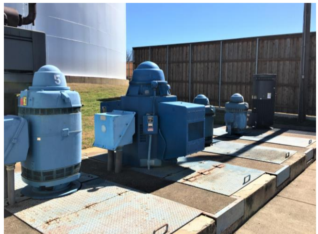
Figure 2.6. High Service Pumps
