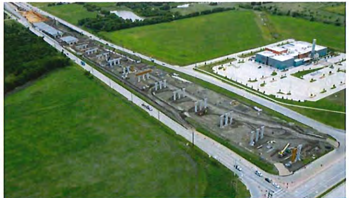
Looking south at the bridge being constructed near US 380
