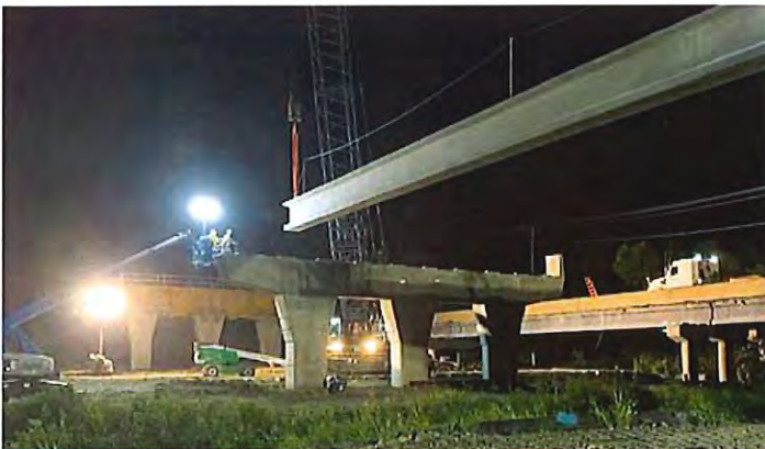
Placing beams at Parvin Branch Creek
