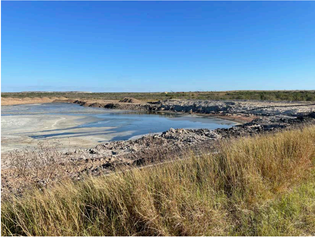
Photograph 9: View of southern berm of EQ Pond half cut, looking southeast.
