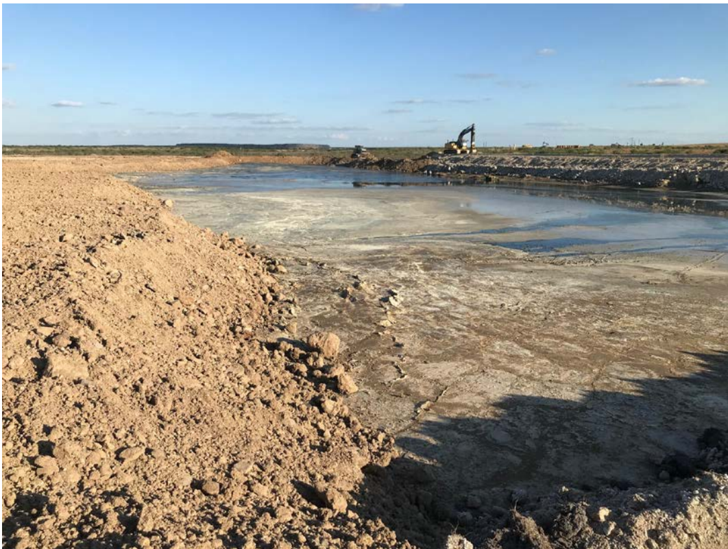
Photograph 10: View of southern berm of EQ Pond being cut, looking southeast.
