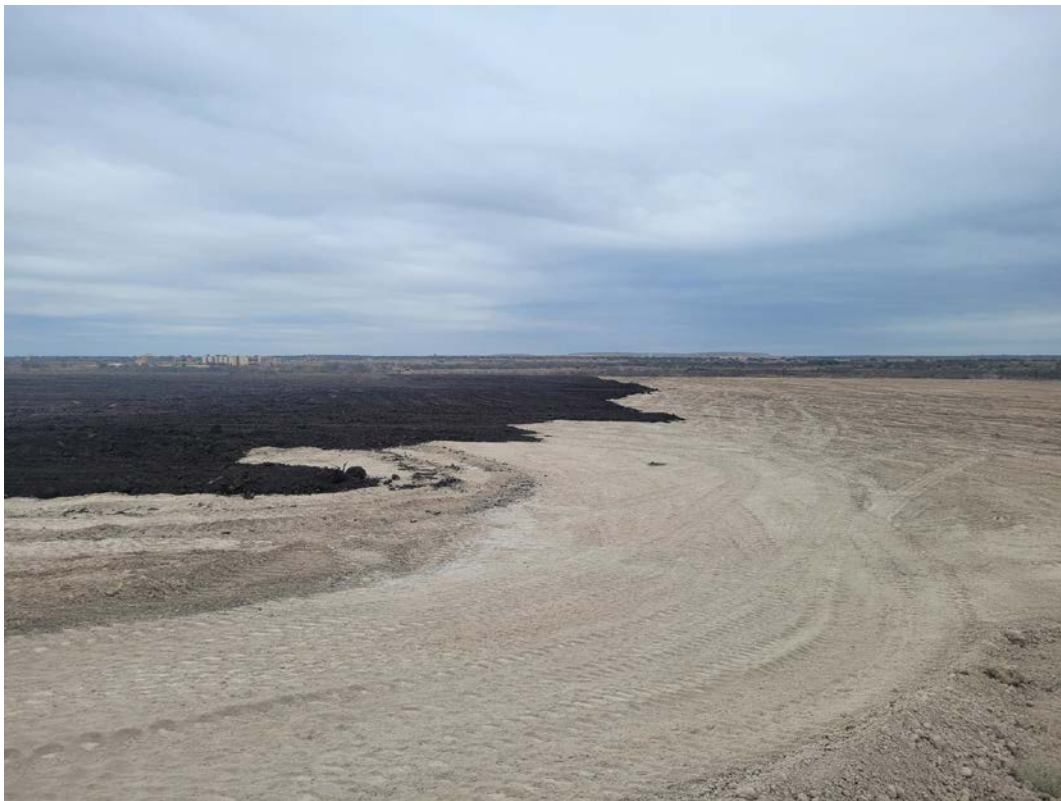
Photograph 14: View of top soil laid out over EQ Pond cap, looking east.
