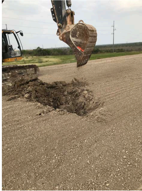
Photograph 13: View of test pit dug in EQ Pond cap, looking northeast.
