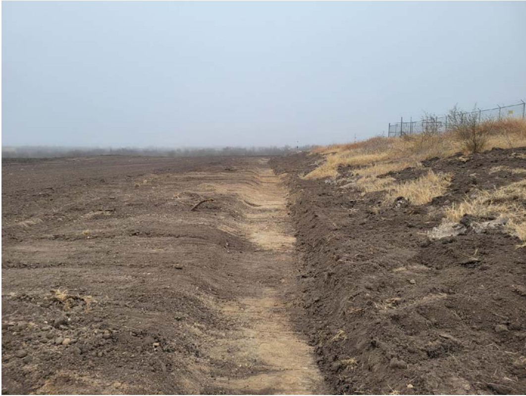
Photograph 15: View of drainage swale construction, looking south.
