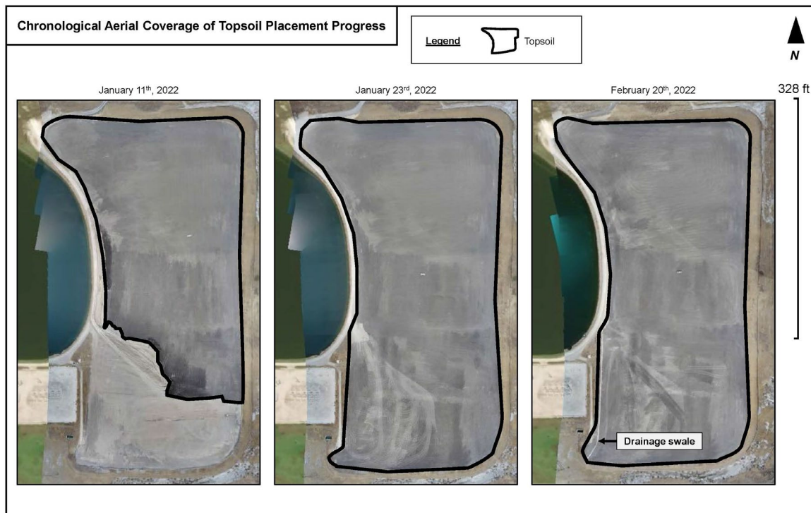
Figure 8 Chronological Aerial Coverage of Topsoil Placement Progress
