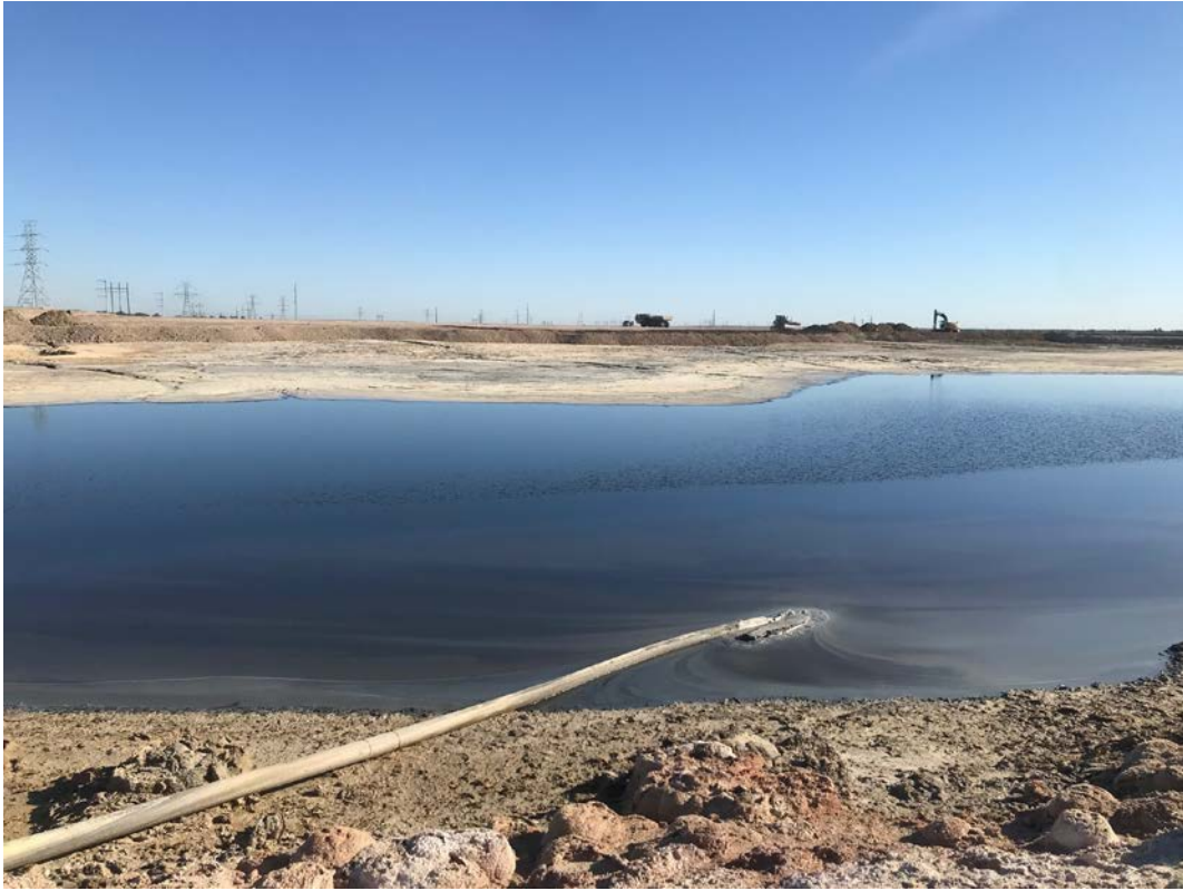
Photograph 11: View of water being pumped out of EQ Pond, looking east-northeast.
