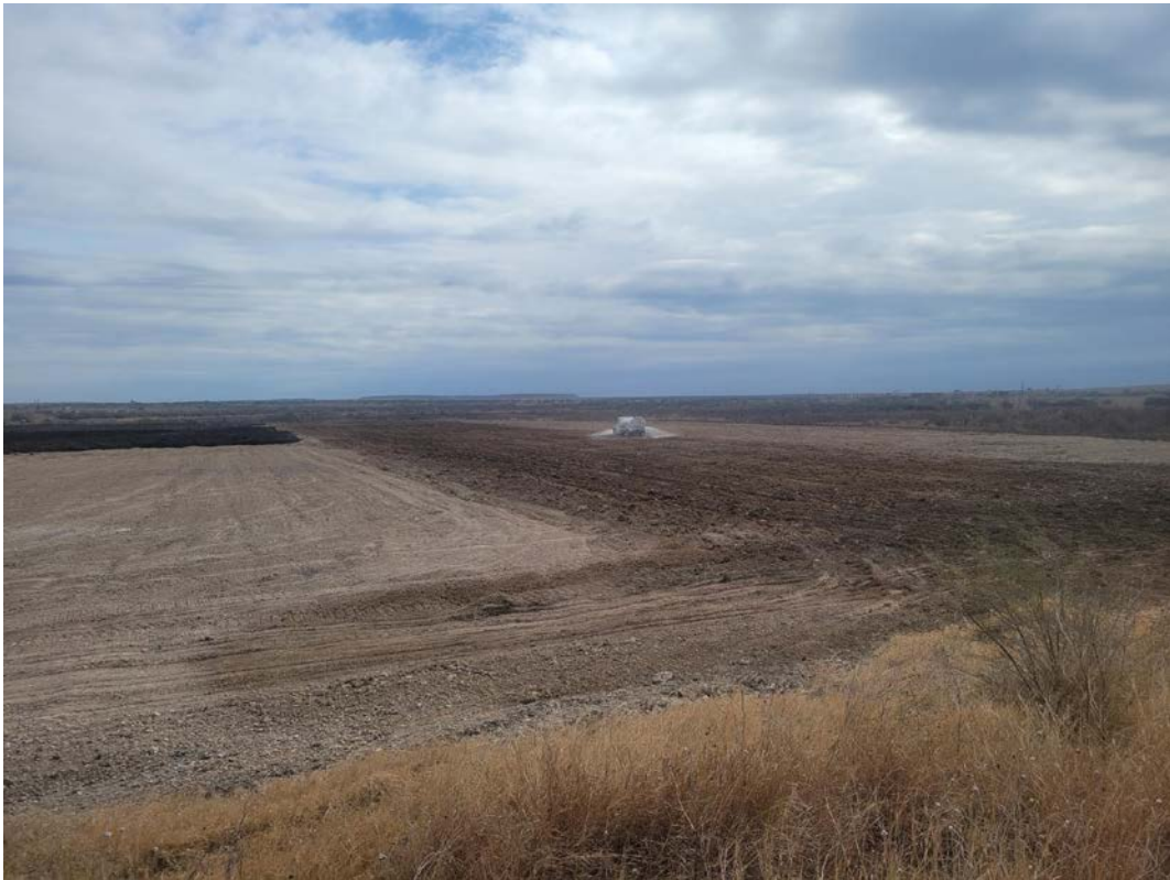
Photograph 12: View of ripped section of EQ Pond being wetted, looking southeast.
