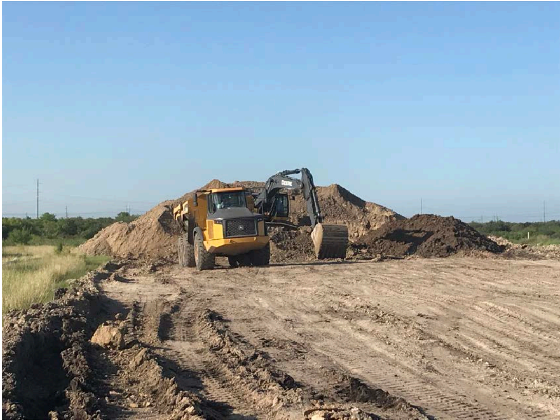
Photograph 1: View of clay stockpile area looking south.
