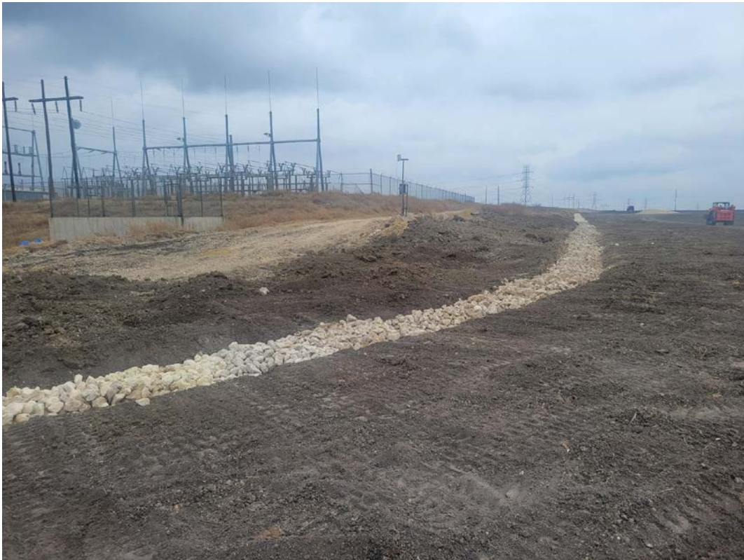
Photograph 16: View of completed drainage swale, looking north.
