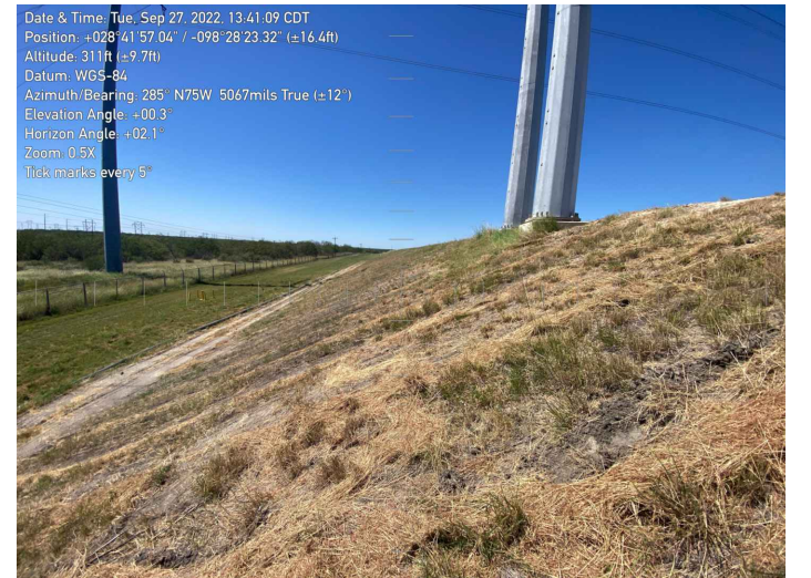
7338 - Facing West. Ash Pond B, South Exterior Slope.
