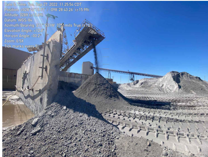
7200 - Facing Southwest. Ash Pile and Wall.
