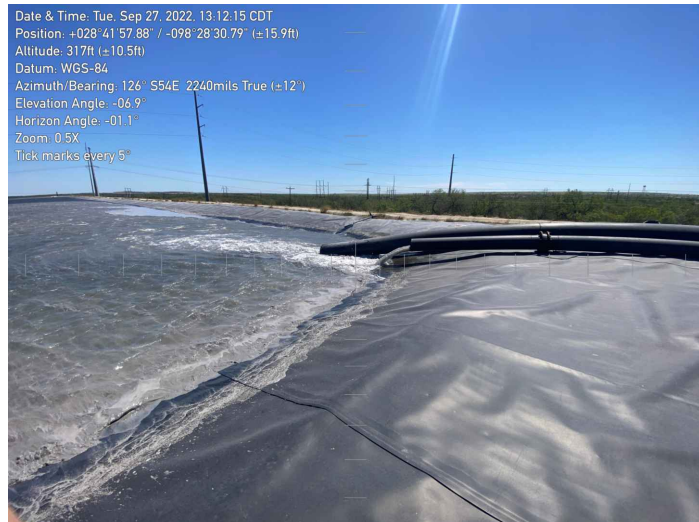
7302 - Facing Southeast. Ash Pond B Splitter Dike.
