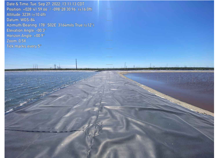
7296 - Facing South. Ash Pond B and South Equalization Basin Splitter Dike.
