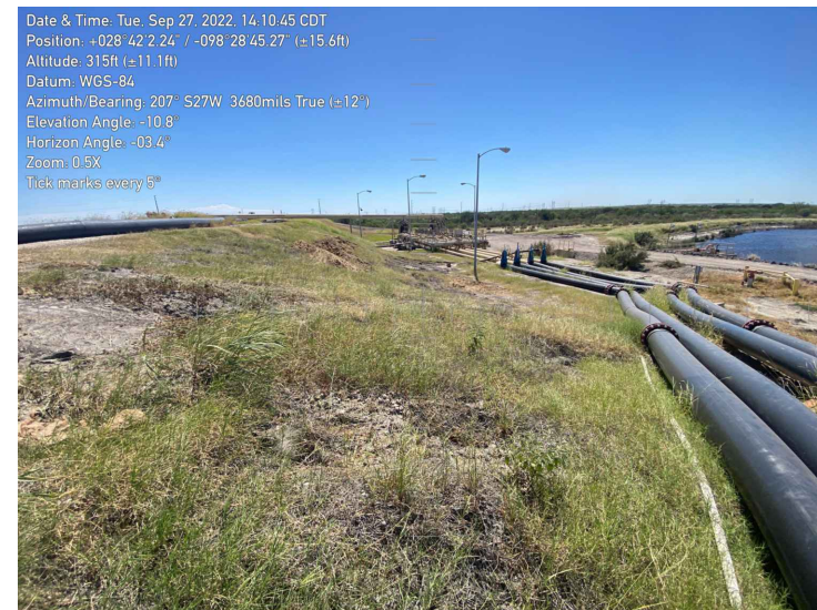
7360 - Facing South. Ash Pond A, West Exterior Slope.
