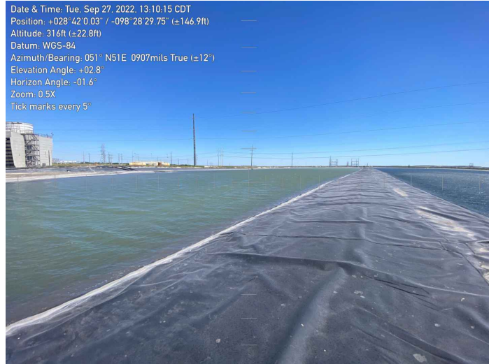
7284 - Facing East. Ash Pond A and South Equalization Basin Interior Dike.
