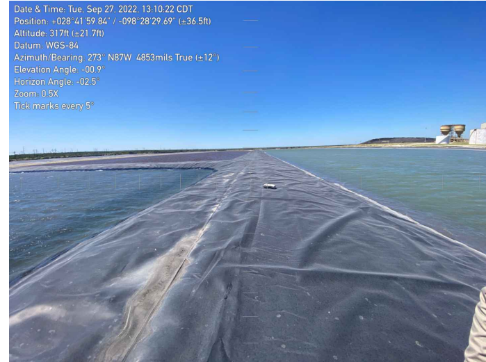
7292 - Facing West. Ash Pond A and Ash Pond B, Interior Dike.
