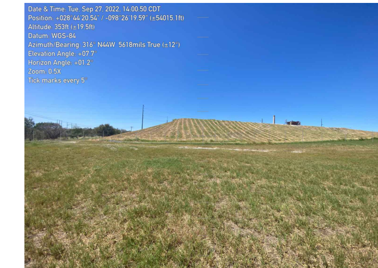
7348 - Facing West. Ash Pond B Exterior.
