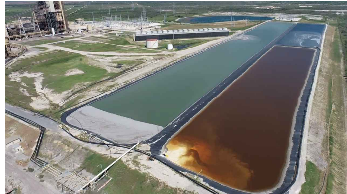
7285 - Facing Northeast. Aerial view of ponds.
