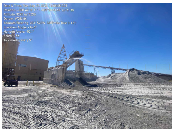
7273 - Facing West. Ash Pile and Sprinklers.
