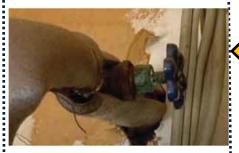
Interior water shut off valves are located under the sinks, and on the side of your toilets. Turn the valves clockwise to shut them off.
