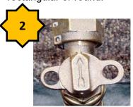
There is a single valve in the meter box. To turn the water off, use a wrench to turn the valve one half turn clockwise until the arrow faces away from the meter. Turn the water back on, turn it one half turn back toward the meter.
