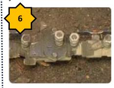
Inside the box is a series of cut-off valves on each end. Either of the valves will shut off the water to your irrigation system.
