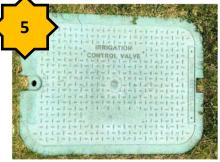
The irrigation valve box is green and typically located near the exterior shut-off of your home near the water
