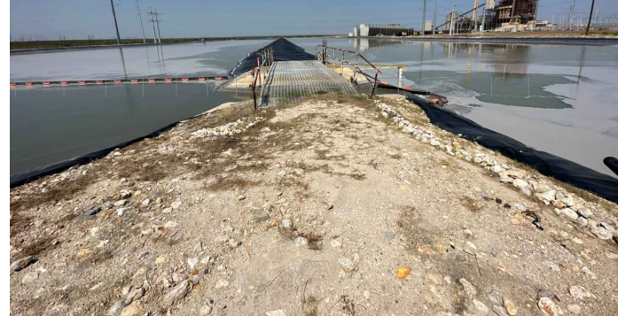
9123 - Facing West. Ash Pond A and Ash Pond B Dike Crest.
