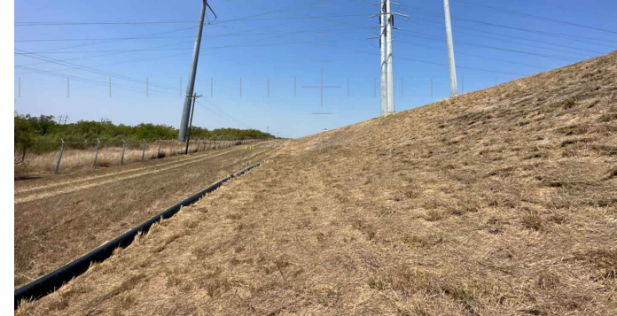
9150 - Facing West. Ash Pond A, South Exterior Slope.
