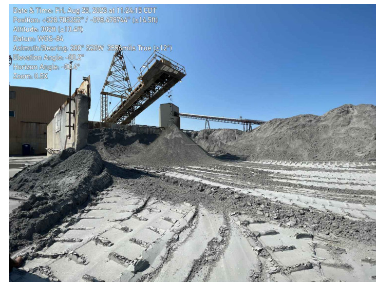
9060 - Facing Southwest. Ash Pile and Wall.
