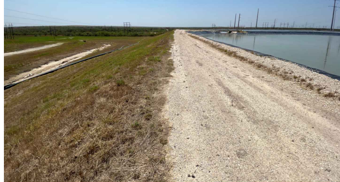
9120 - Facing South. Ash Pond A and Ash Pond B Dike Crest.
