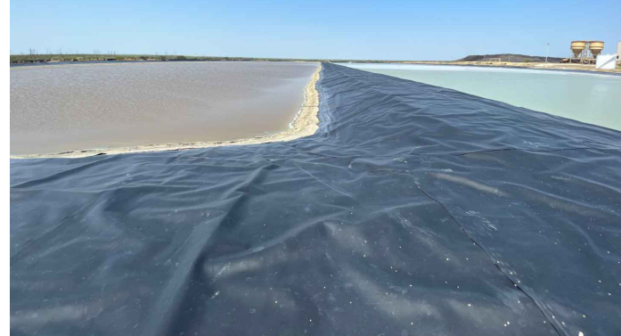
9165 - Facing West. South Equalization Basin, Splitter Dike.
