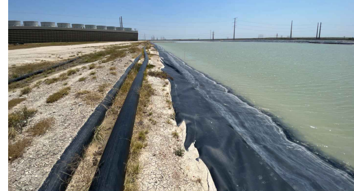
9170 - Facing East. Ash Pond A, Dike Crest.
