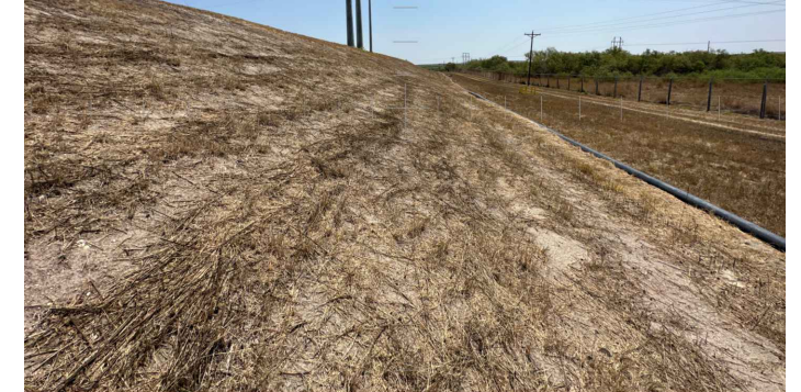
9151 - Facing East. Ash Pond A, South Exterior Slope.
