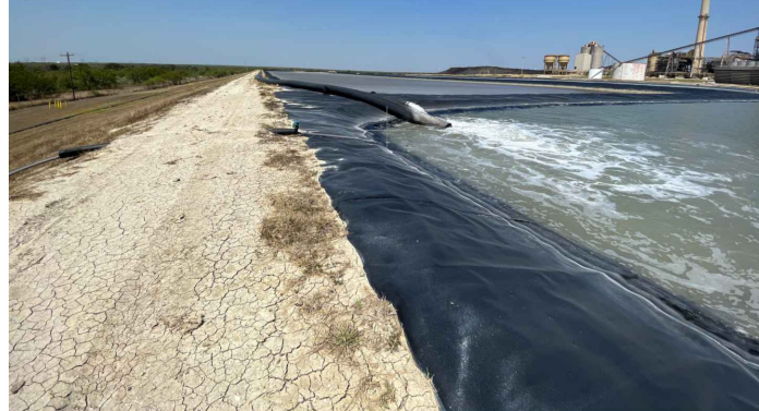
9160 - Facing West. Ash Pond B Splitter Dike.
