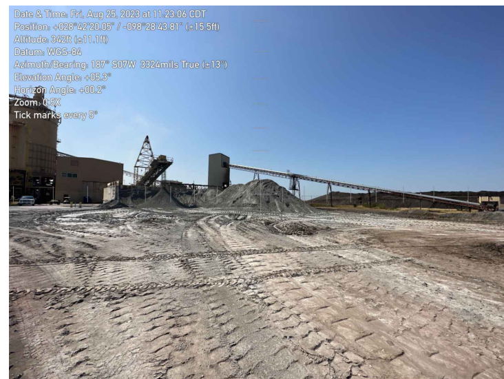
9055 - Facing South. Ash Pile and Wall.
