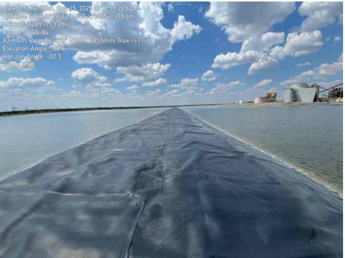
1629 - Facing West. Splitter Dike Crest Between Ash Pond A (right) and Ash Pond B (left)
