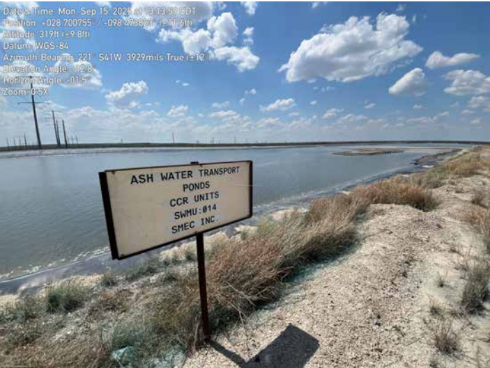
1609 - Facing Southwest. Ash Pond A Exterior Slope and Typical Signage.
