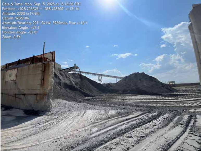
1801 - Facing Southwest. Ash Pile and Wall.
