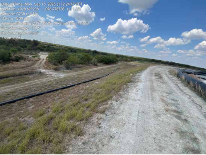
1653 - Facing Southwest. SEB Dike Crest and Exterior Slope
