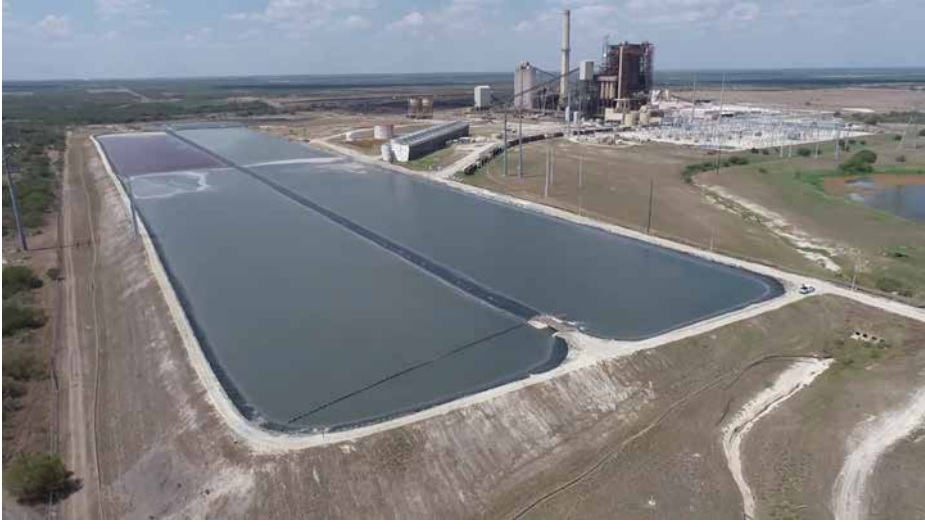
1701 - Facing Northwest. Ash Ponds and SEB, Aerial Overview
