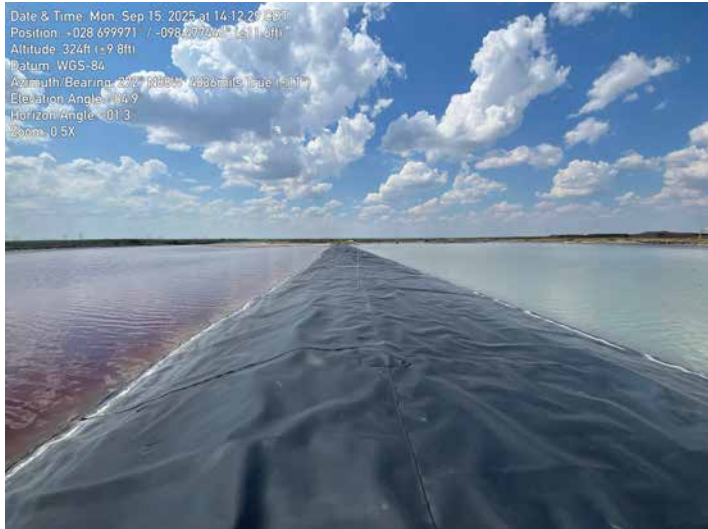
1637 - Facing West. Ash Pond B and SEB Splitter Dike Crest.
