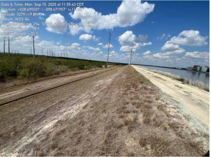
1647 - Facing Southwest. Ash Pond B, Dike Crest and Exterior Slope.
