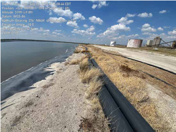
1603 - Facing West. Ash Pond A Northern Dike.
