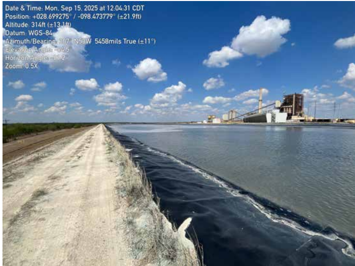
1641 - Facing Northwest. Ash Pond B, Interior Slope (right) and Exterior Slope (left)
