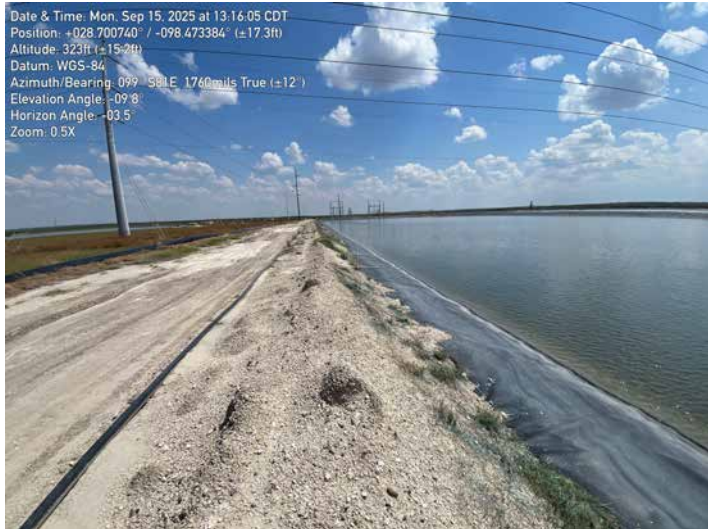
1615 - Facing Southeast. Ash Pond A Interior Slope (right) and Exterior Slope (left).
