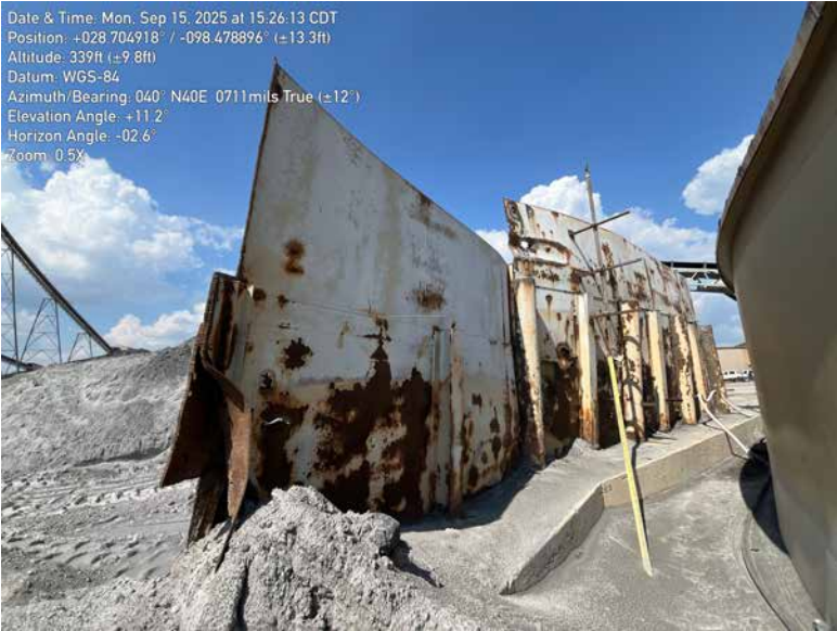
1809 - Facing Northeast. Ash Pile Wall.
