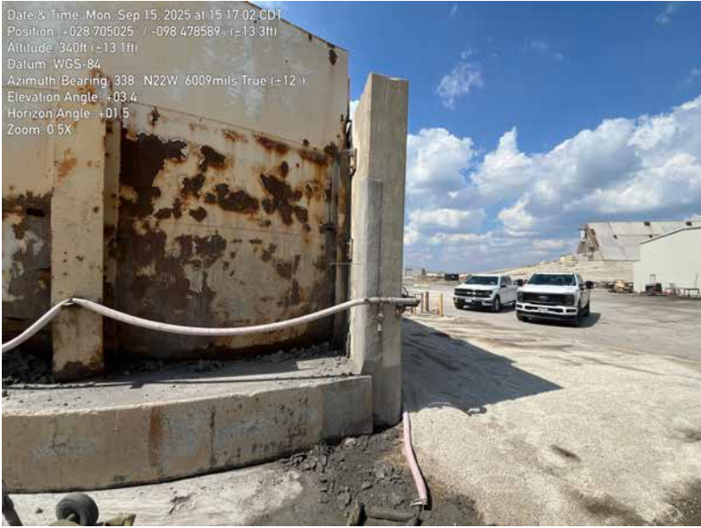
1811 - Facing Southeast. Ash Pile Wall.
