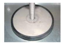
2 Placing of the sealing disc
