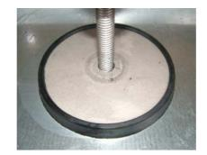
**2nd step** Place the sealing disc.
