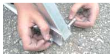
② Screw the module beam
