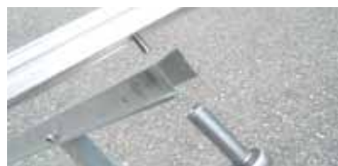
③ Mount the module beam
