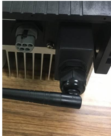
Fig. Complete the installation
