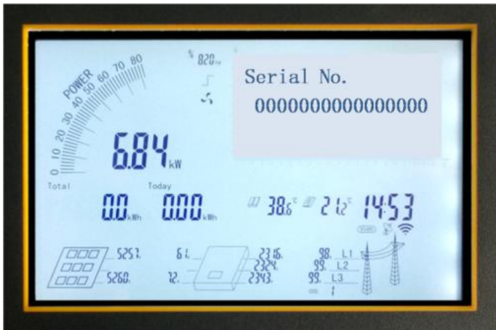
Figure 33 Inverter SN interface
