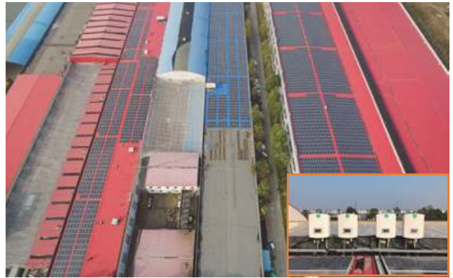
Shandong Weifang Linqu poverty alleviation PV Plant 20MW
