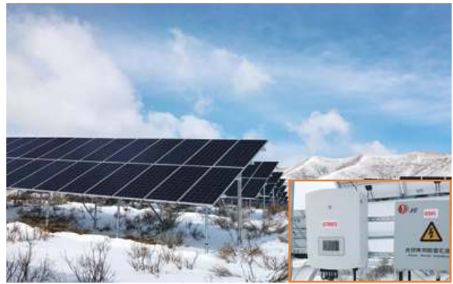
Shanxi Guangling PV plant 1.47MW
