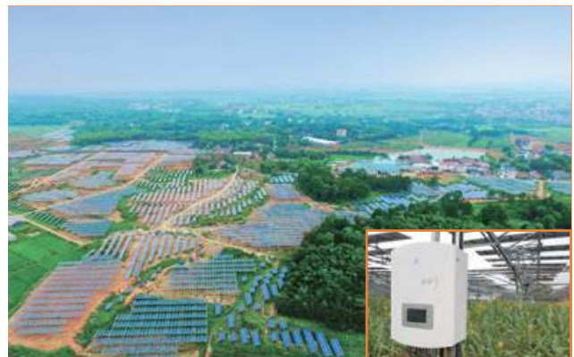
Quzhou Qinghu Agricultural-photovoltaic hybrid PV plant 20MW
