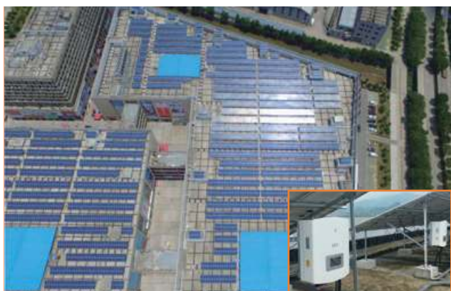
Ninghai AB hall, modern home plaza 1.53MW
