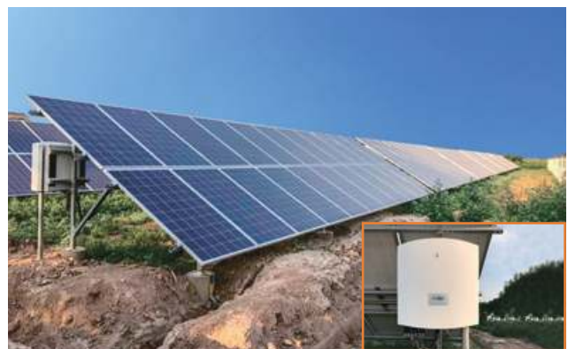
Hebei Qinghuangdao poverty alleviation PV Plant 5MW
