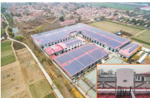
Shandong YUELONG 3.5MW
