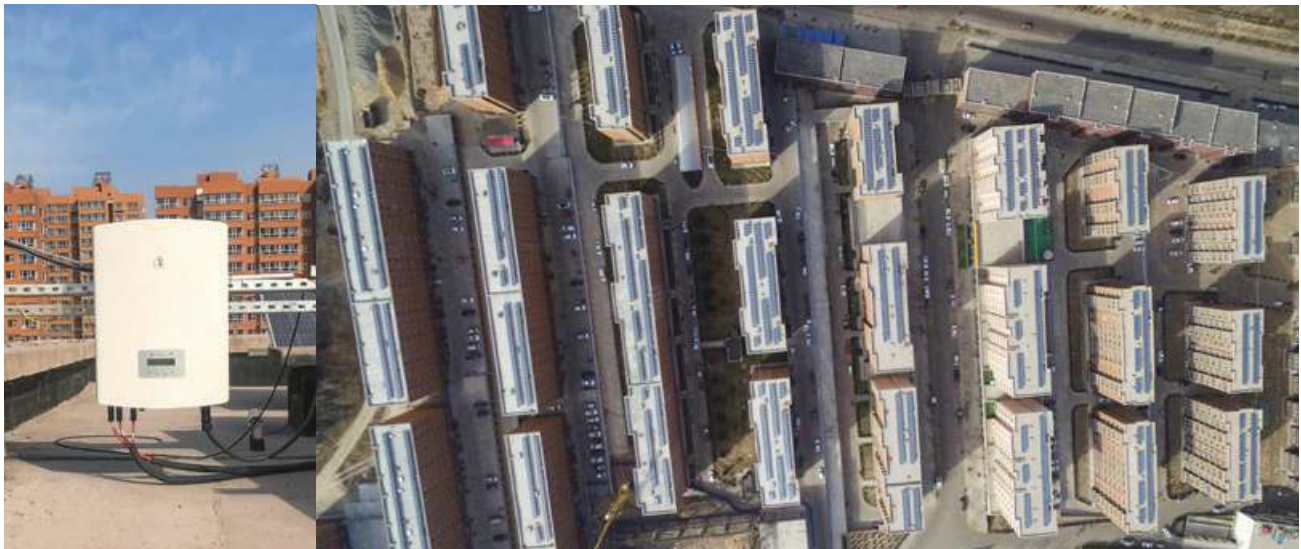
Shanxi Lvliang ZhongYang Jiajingtiancheng PV rooftop 450kW
