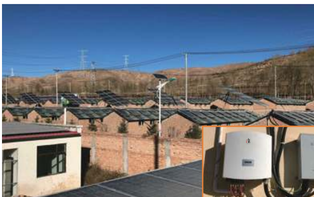
Qinghai HuzhuBanyan poverty alleviation PV Plant 2MW
