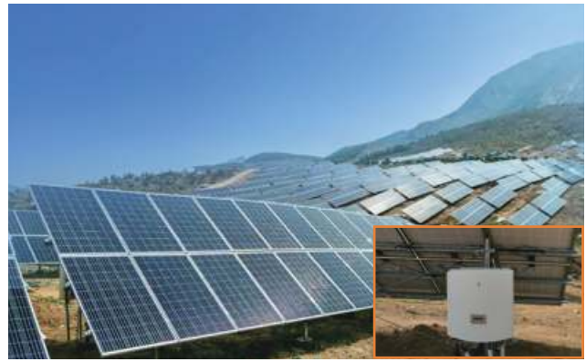
Liaoning Yingkou Jiuzhai PV plant 20MW
