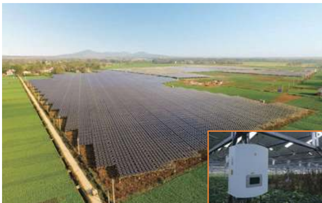
Hubei Guanyin Agricultural-photovoltaic hybrid PV plant 20MW
