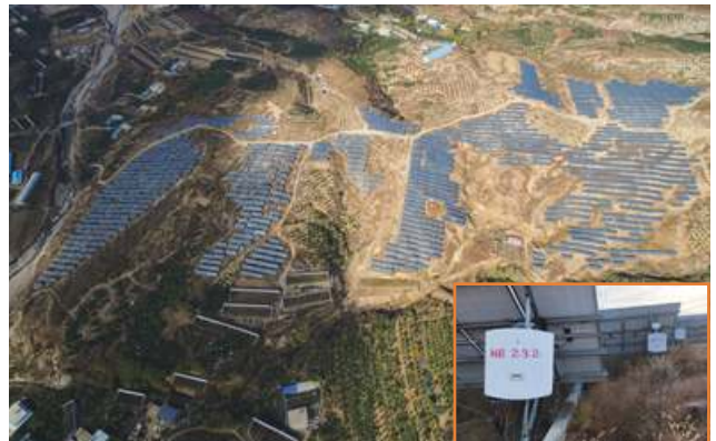
Liaoning Jiuzhai Gaizhou PV plant 20MW
