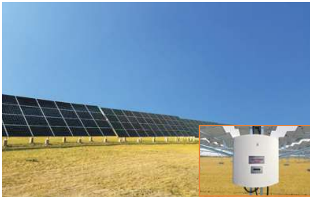
Huaneng Yimin surface mine PV plant 20MW
