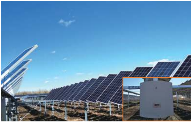
Hebei Zhangbei Agricultural-photovoltaic hybrid PV plant 50MW
