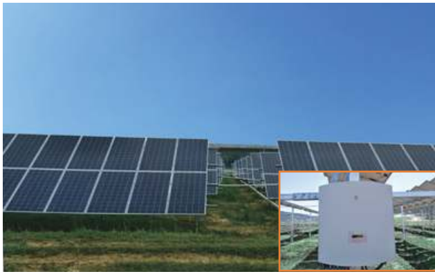
Hebei Zhangjiakou poverty alleviation PV Plant 5.1MW
