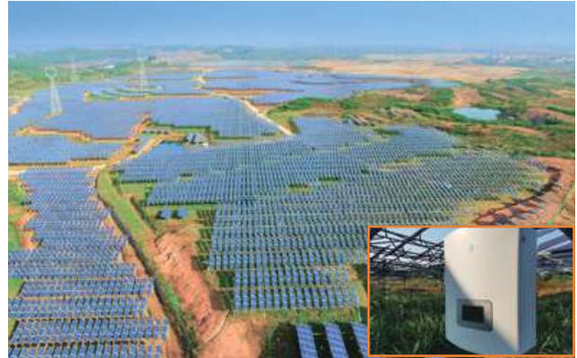
Zhejiang Hangbu Agricultural-photovoltaic hybrid PV plant 30MW
