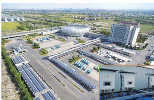
Zhejiang PINGHU Bus Station 472kW
