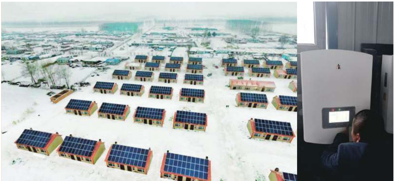
Heilongjiang PV plant
