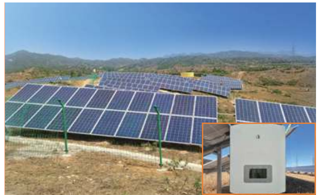
Hebei Qinghuangdao poverty alleviation PV Plant 9.7MW
