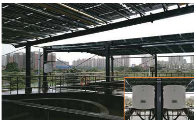
Hunan Yongzhou dao county water plant 800kW
