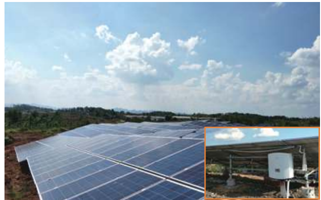
Jiangxi Ganzhou PV Plant 3.5MW
