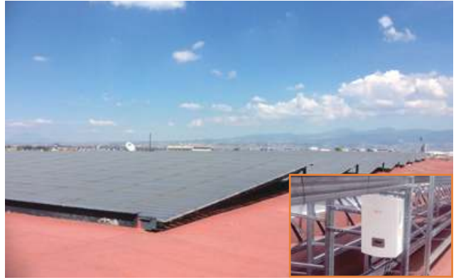
Mexico Soccer Federation 180kW
