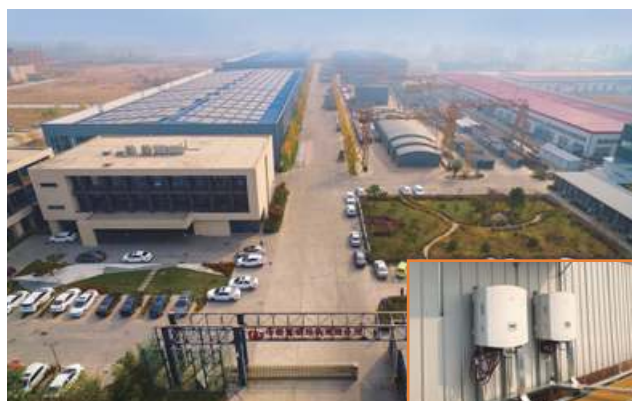
Hebei ZQ Steel 1.5MW
