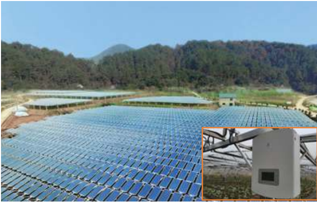
Zhejiang Dajie Agricultural-photovoltaic hybrid PV plant 3MW
