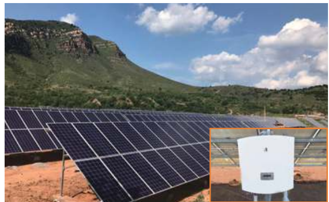
Shanxi Xiyang poverty alleviation PV Plant 7.2MW
