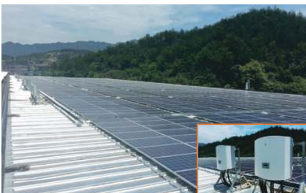
Hainan JiuLongGlass 1.7MW
