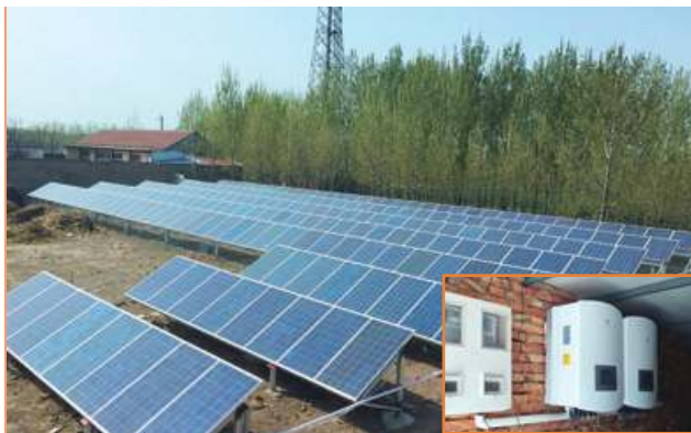
Shandong Leling poverty alleviation PV Plant 50kW
