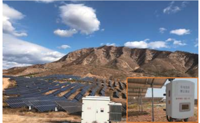
Liaoning Gaizhou Jiuzhai PV plant 20MW
