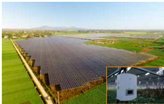
Hubei Guanyin Agricultural-photovoltaic hybrid PV plant 20MW
