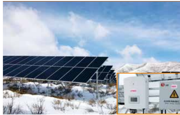
Shanxi Guangling PV plant 1.47MW
