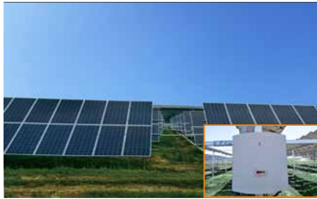
Hebei Zhangjiakou poverty alleviation PV Plant 5.1MW
