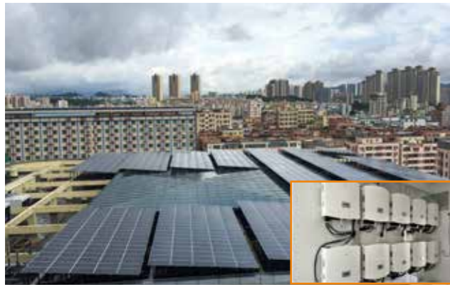
Shenzhen Jiangnan Times Building 600kW
