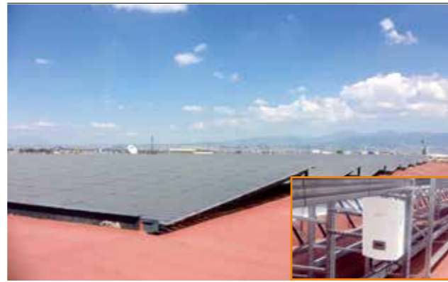
Mexico Soccer Federation 180kW
