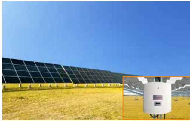
Huaneng Yimin surface mine PV plant 20MW
