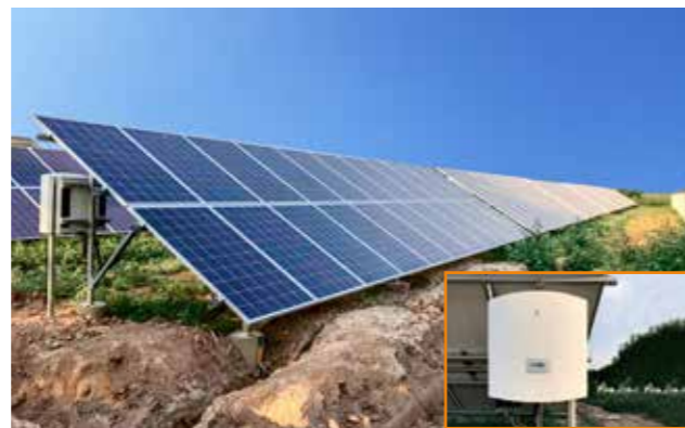
Hebei Qinghuangdao poverty alleviation PV Plant 5MW
