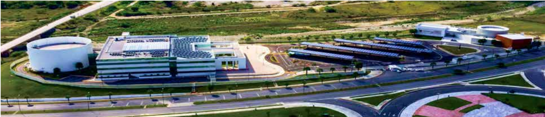
Mexico-Tamaulipas Carport 5MW
