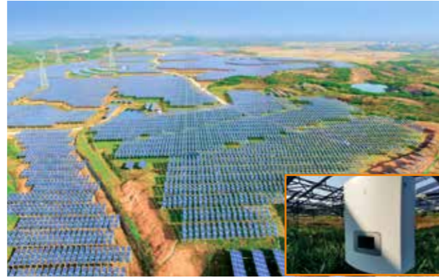
Zhejiang Hangbu Agricultural-photovoltaic hybrid PV plant 30MW
