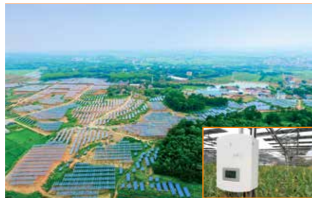
Quzhou Qinghu Agricultural-photovoltaic hybrid PV plant 20MW
