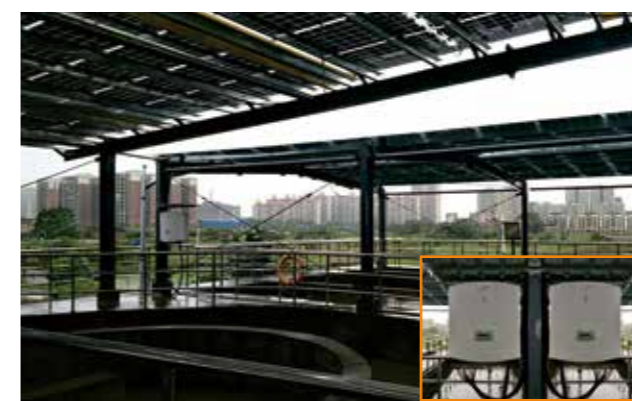
Hunan Yongzhou dao county water plant 800kW
