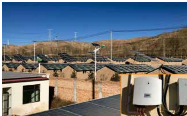
Qinghai HuzhuBanyan poverty alleviation PV Plant 2MW
