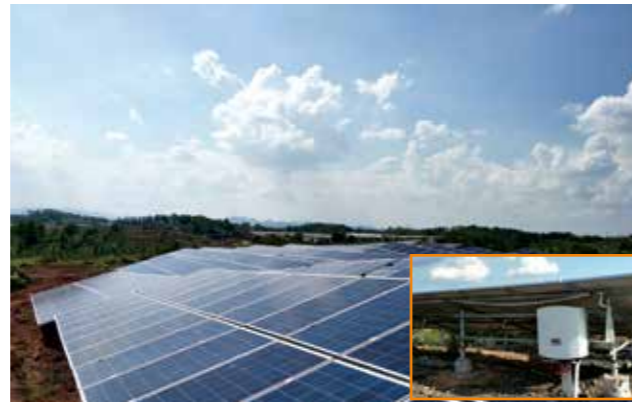
Jiangxi Ganzhou PV Plant 3.5MW
