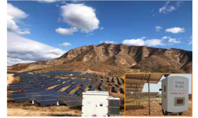
Liaoning Gaizhou Jiuzhai PV plant 20MW
