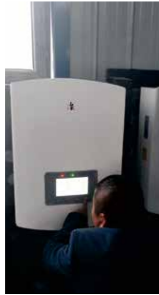
Heilongjiang PV plant
