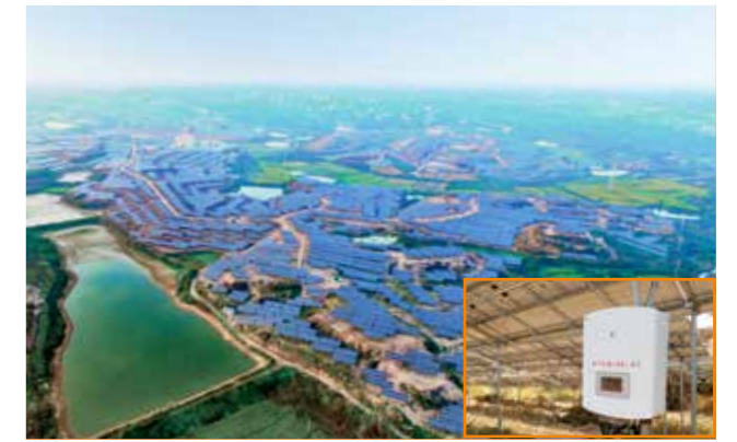
Zhejiang Longyou Agricultural-photovoltaic hybrid PV plant 25MW
