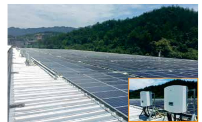
Hainan JiuLongGlass 1.7MW
