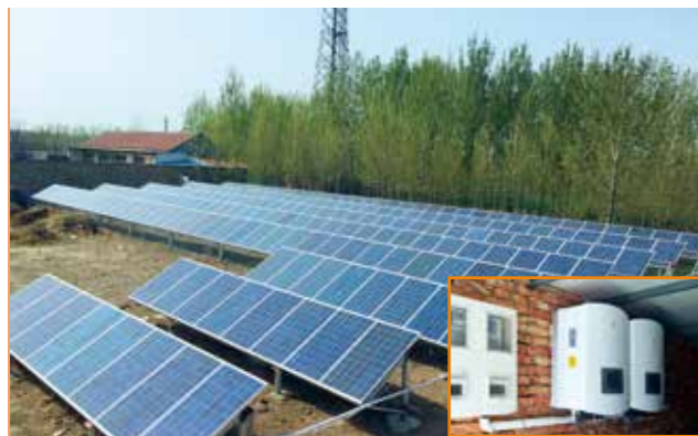
Shandong Leling poverty alleviation PV Plant 50kW
