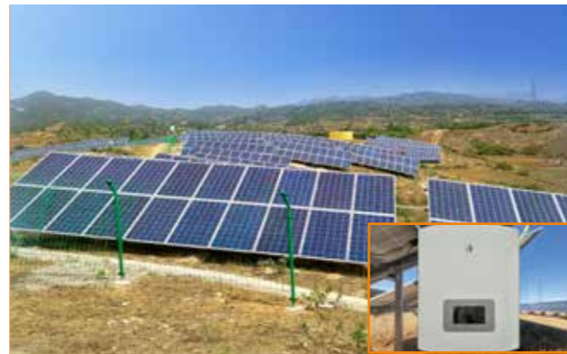
Hebei Qinghuangdao poverty alleviation PV Plant 9.7MW
