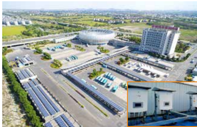
Zhejiang PINGHU Bus Station 472kW
