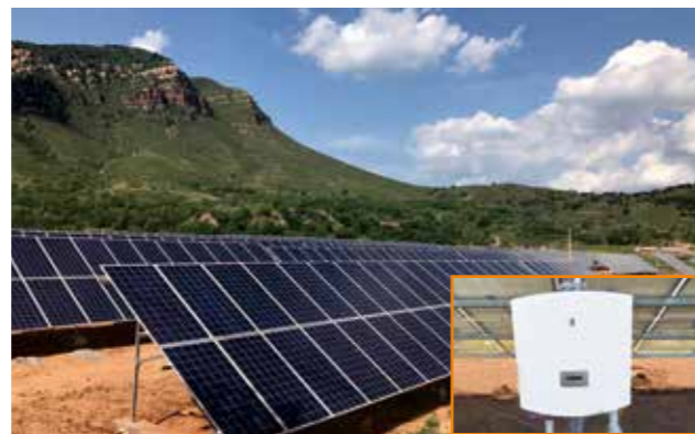
Shanxi Xiyang poverty alleviation PV Plant 7.2MW
