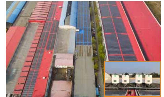
Shandong Weifang Linqupoverty alleviation PV Plant 20MW
