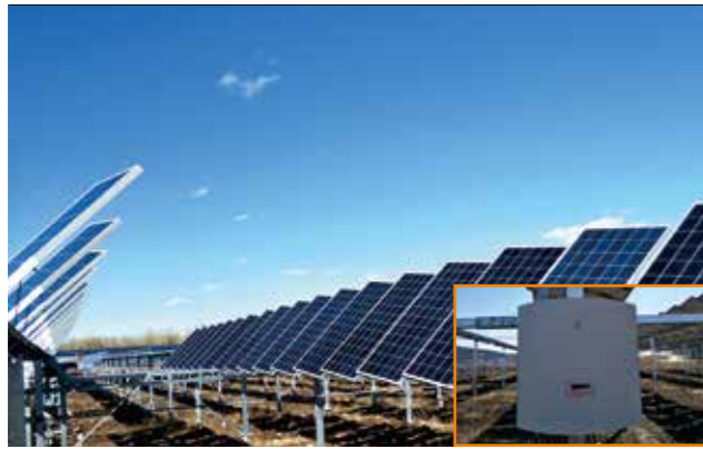
Hebei Zhangbei Agricultural-photovoltaic hybrid PV plant 50MW
