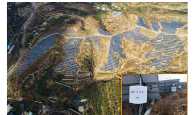
Liaoning Jiuzhai Gaizhou PV plant 20MW
