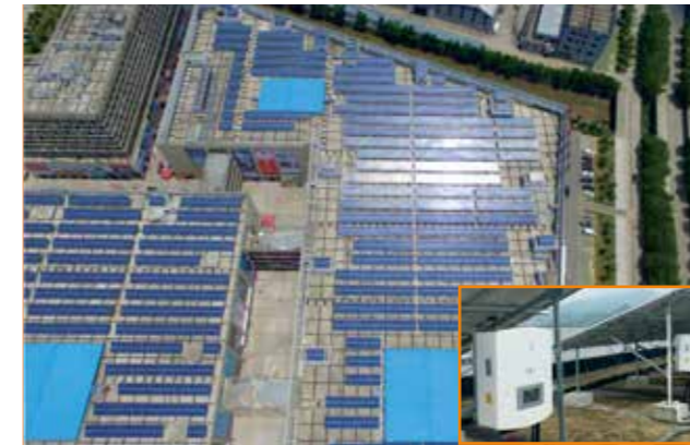
Ninghai AB hall, modern home plaza 1.53MW
