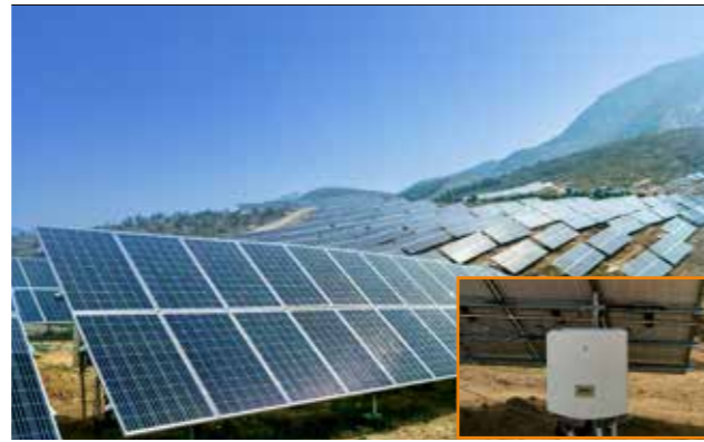
Liaoning Yingkou Jiuzhai PV plant 20MW
