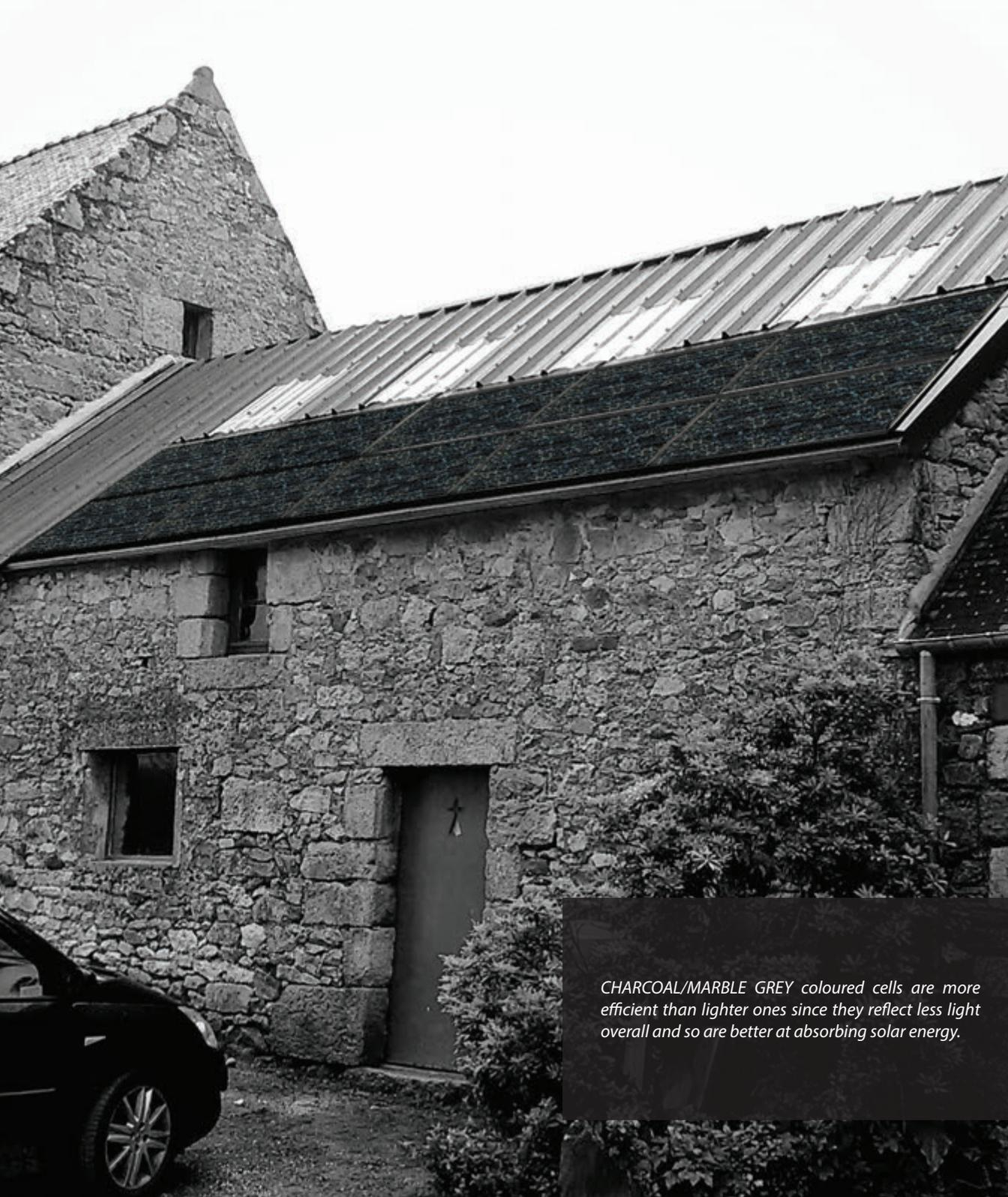
*CHARCOAL/MARBLE GREY coloured cells are more efficient than lighter ones since they reflect less light overall and so are better at absorbing solar energy.*
