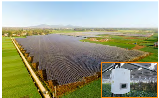
Hubei Guanyin Agricultural-photovoltaic hybrid PV plant 20MW
