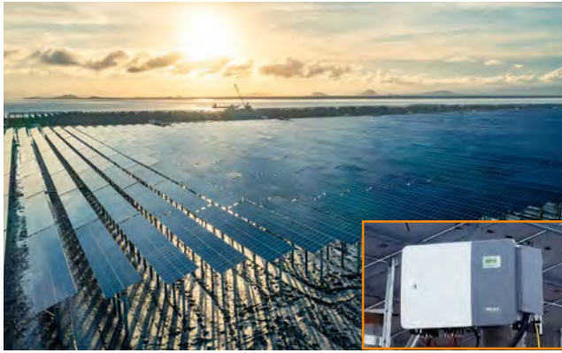
Zhejiang Ningbo Tidal Flat Project 300MW
