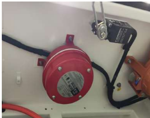
Figure 5-29 Aerosols activated by thermal sensitive wires
