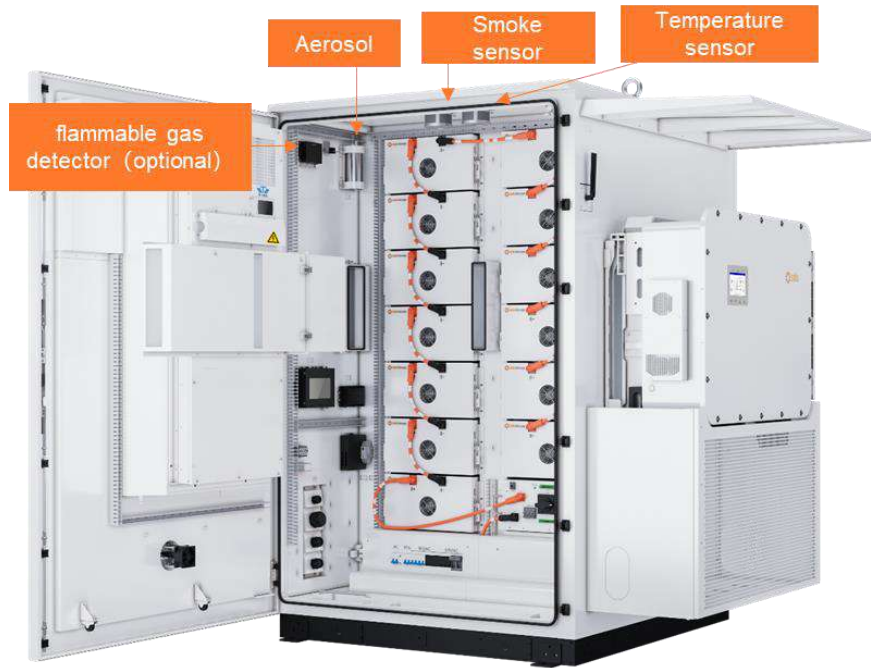
Figure 3-5 Detector Installation Layout
