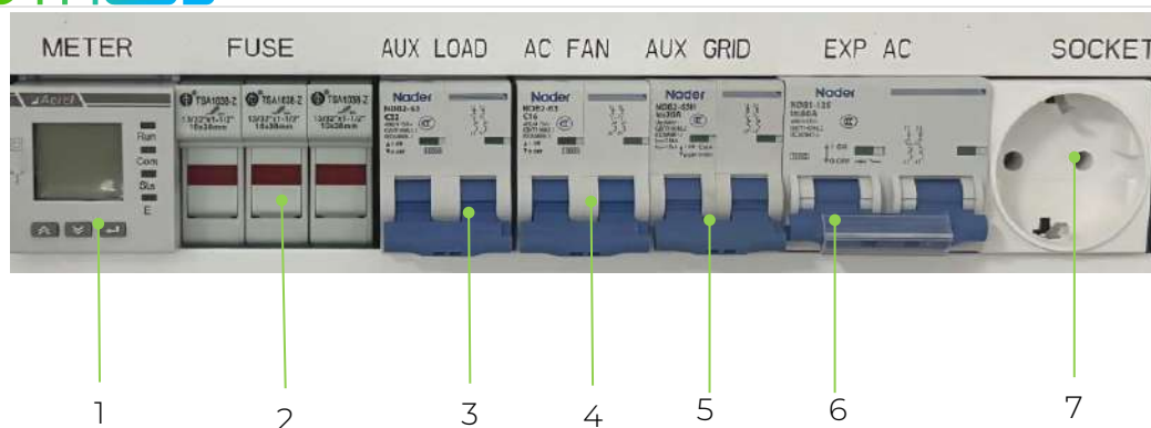
Figure 3-7 Schematic Diagram of Secondary Switches in the Front Electrical Compartment
