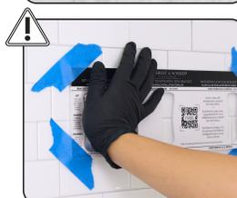
**ÉTAPE 7 : APPUYER FERMEMENT SUR LE SUPPORT** (minimum de 6,8 kg-force)
